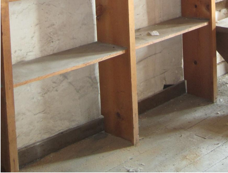
Figure 52. Third Floor: baseboard.
