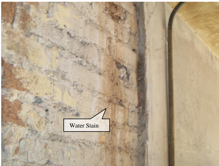
Figure 74. Third Floor: plaster laid over brick.
