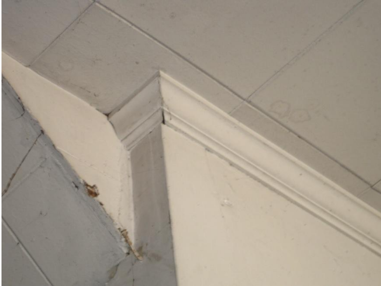
Figure 40. First Floor: crown molding.
