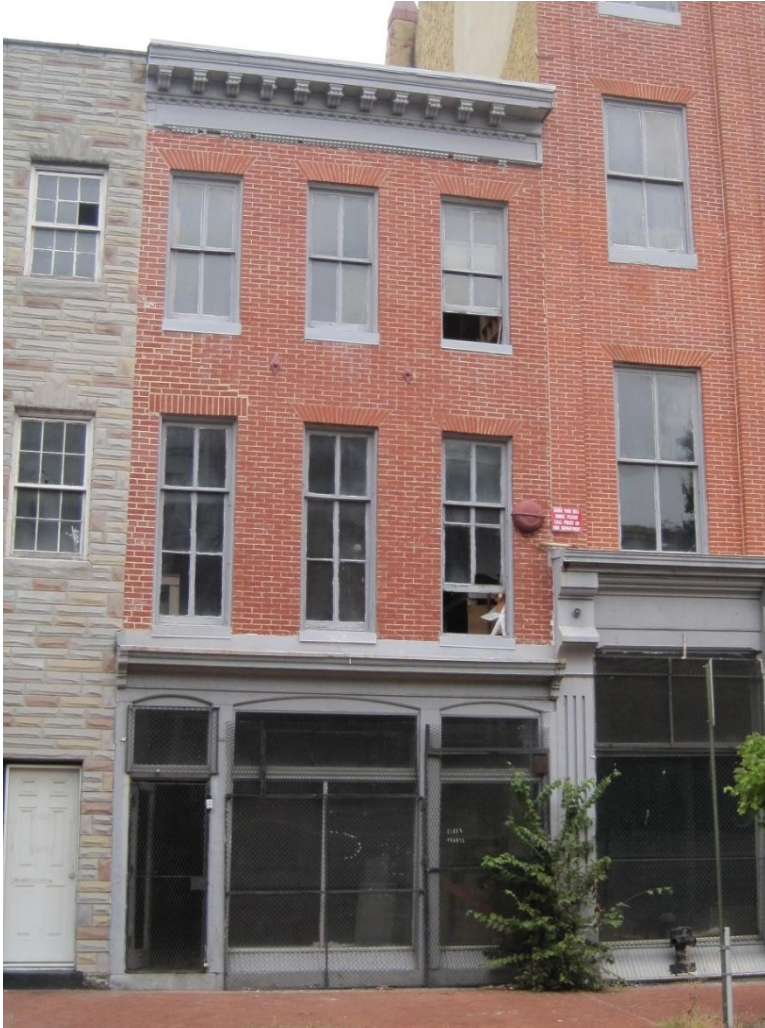
Figure 11. Exterior: south elevation.
