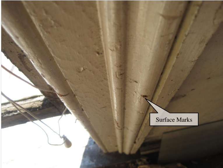
Figure 50. Second Floor: detailed window trim profile and marks in surface.
