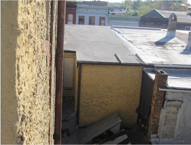
Figure 88. Exterior: flat roof.
