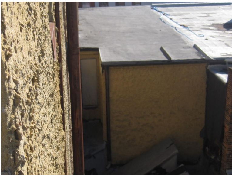
Figure 12. Exterior: north elevation.
