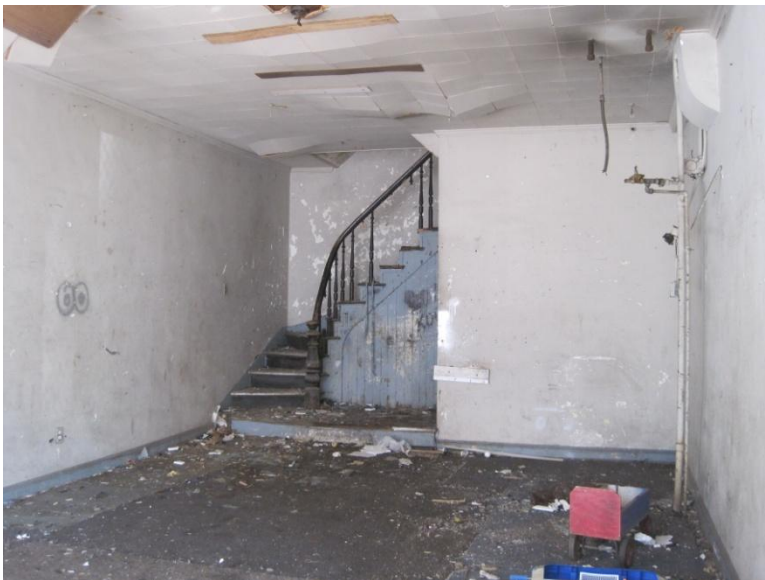
Figure 14. First Floor: north interior elevation.
