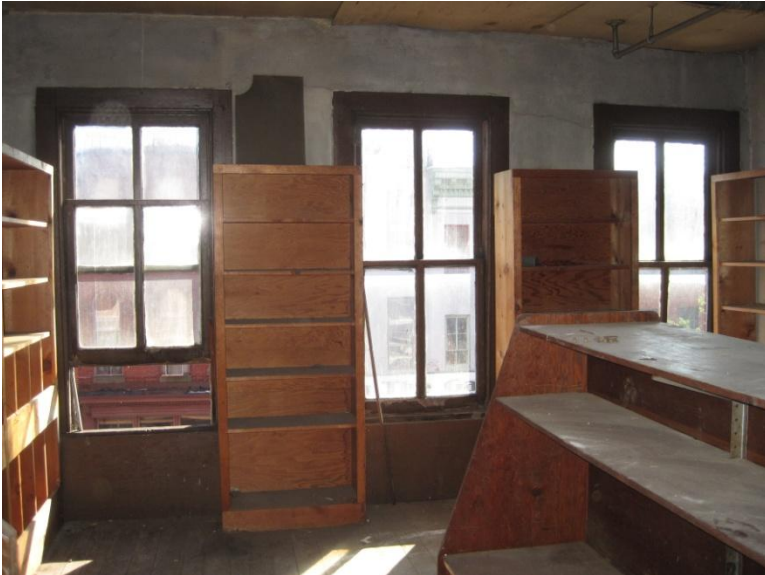
Figure 53. Third Floor: window trim.
