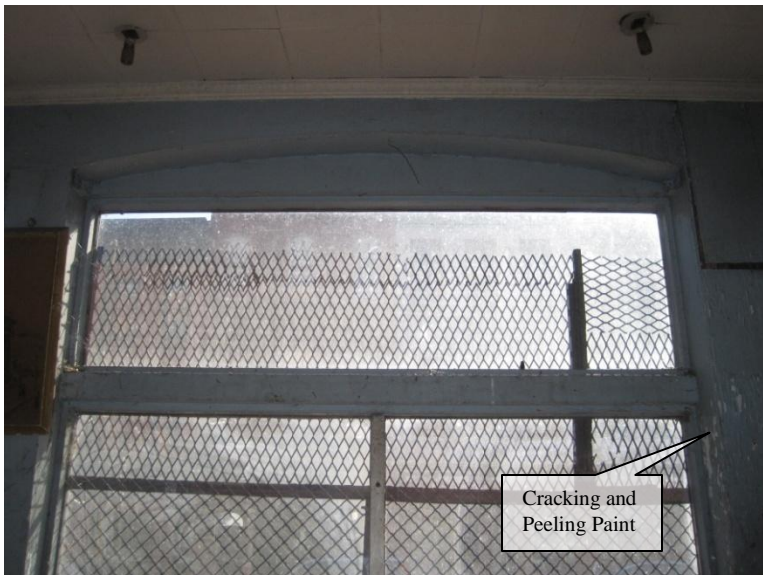
Figure 59. First Floor: storefront windows and transom.
