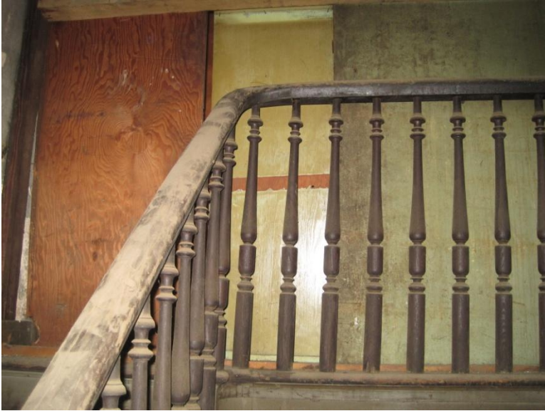
Figure 39. Third Floor: best preserved handrail and balusters.
