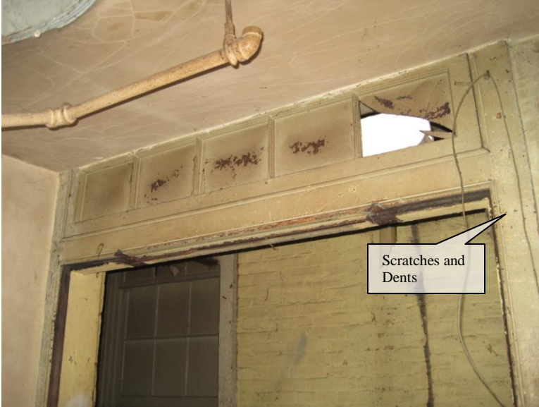
Figure 43. First Floor: doorway and transom trim under the stair.
