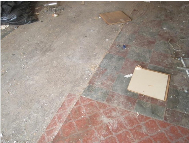
Figure 72. Second Floor: plywood subflooring and two layers of vinyl tile.
