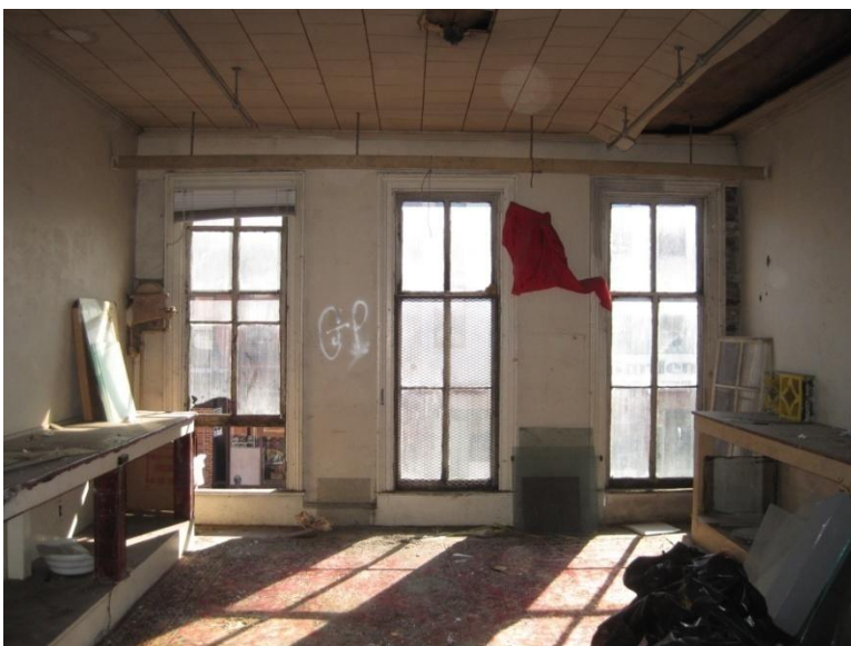
Figure 15. Second Floor: south interior elevation.
