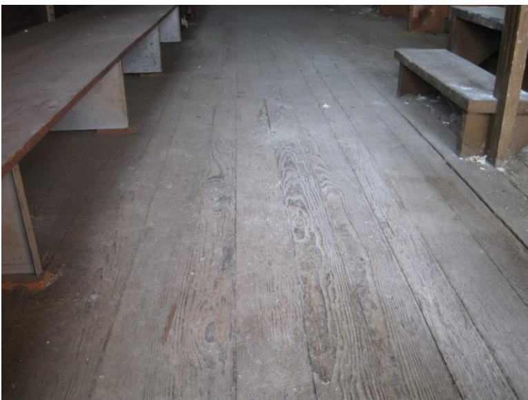
Figure 73. Third Floor: random width wood floor boards.
