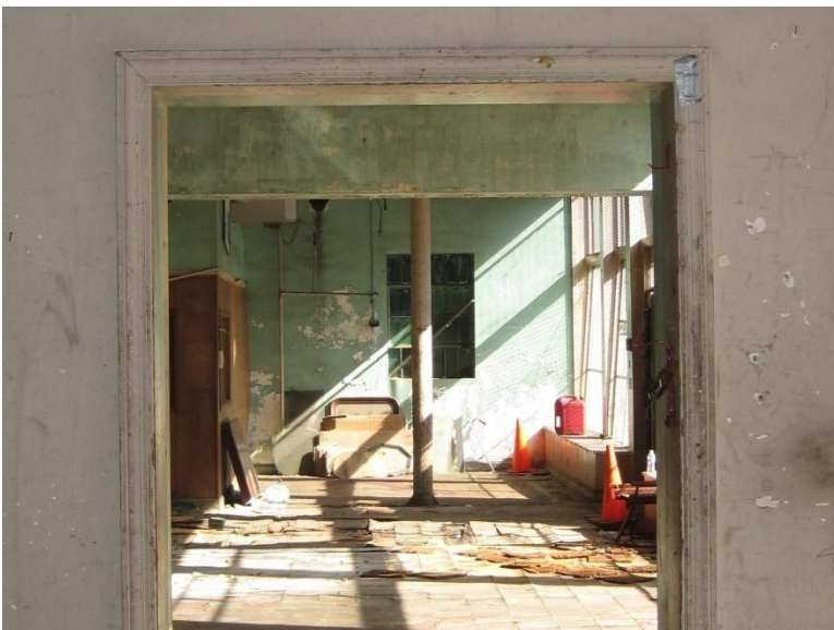
Figure 42. First Floor: east wall doorway trim.
