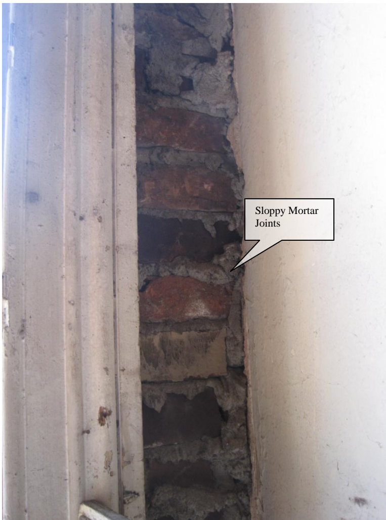
Figure 24. Second Floor: exposed masonry on south wall.
