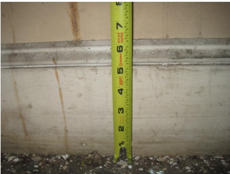
Figure 47. Second Floor: baseboard.
