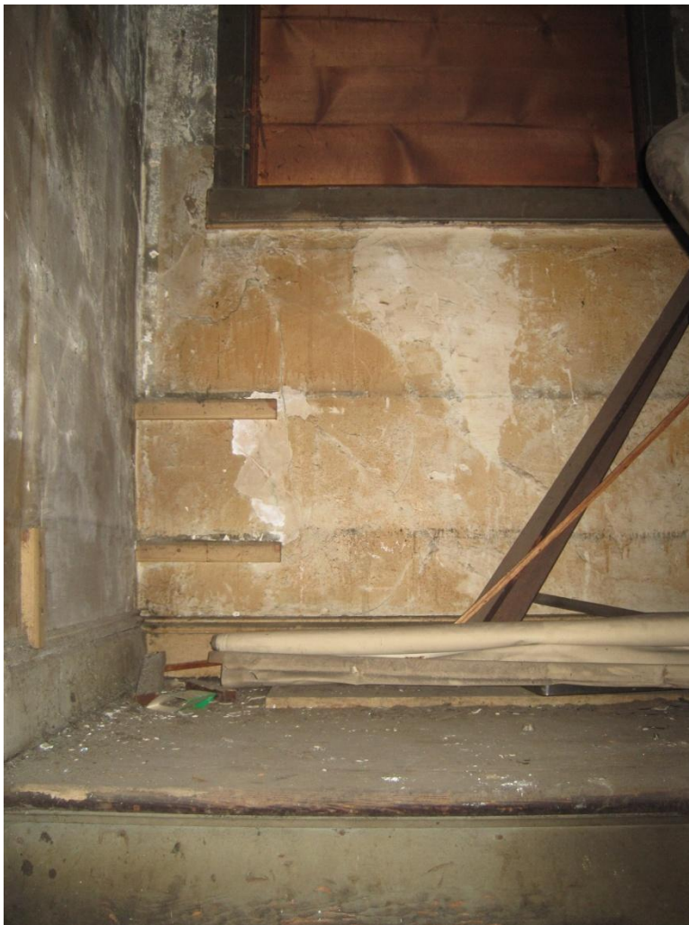
Figure 51. Second Stair Landing: baseboard and window trim.
