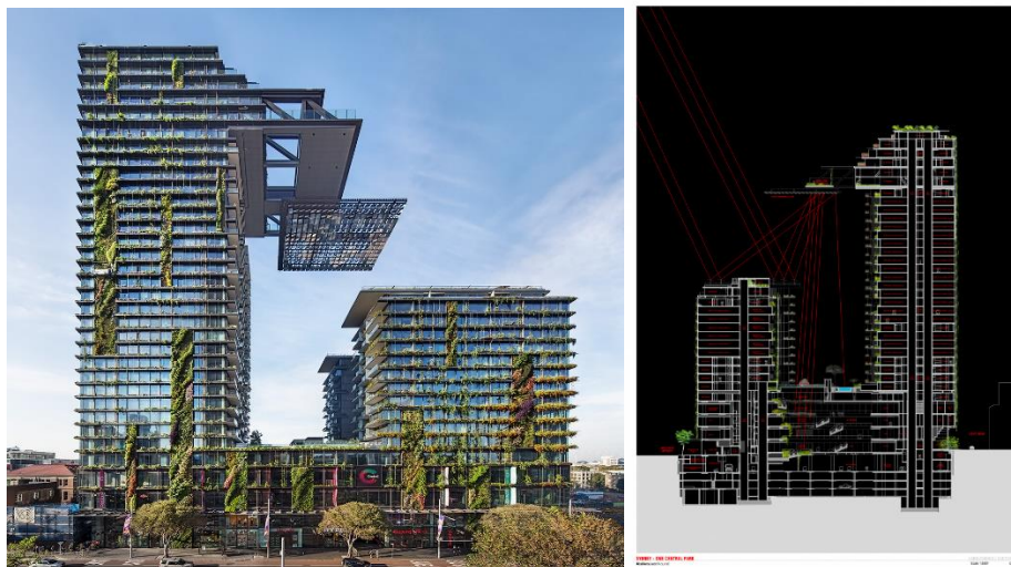
Figure 5.26: Cantilever and Heliostat, photo by Murray Fredericks, drawing by Ateliers Jean Nouvel, ArchDaily, 2014
