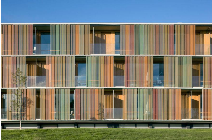
Figure 5.29: Perforated, operable, colored metal screens, photo by Duccio Malagamba, ArchDaily, 2009
