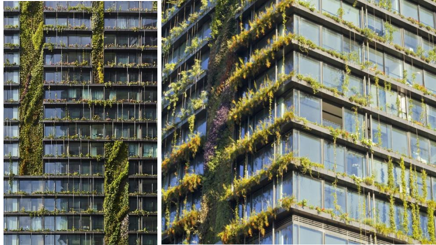
Figure 5.25: Hydroponic growing façade, photos by Murray Fredericks (left) and Simon Wood (right), ArchDaily, 2014
