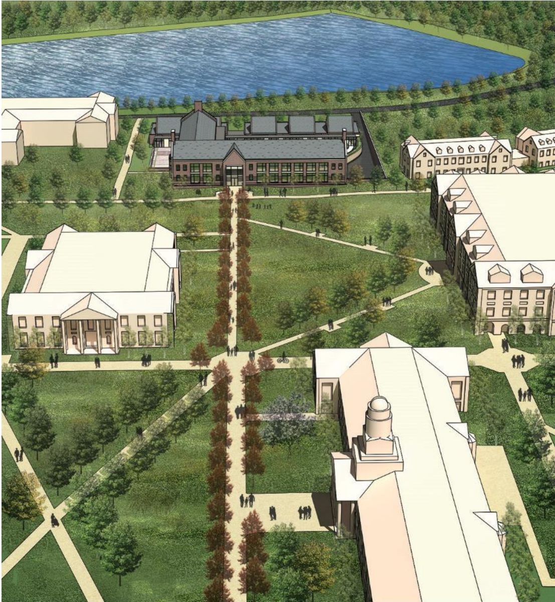
Figure 7.35: Aerial view of building (image by author)
