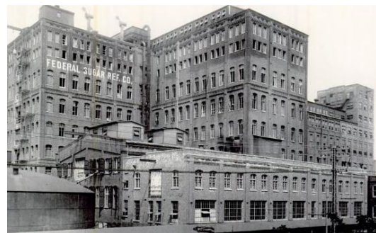
Figure 20: National Sugar Refinery (1863) Credit: Yonkers Historical Society
