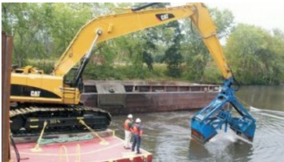
Figure 7: Dredging of the Hudson River Credit: Clearwater.org
