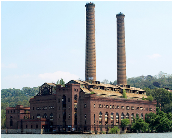
Figure 49: Glenwood Power Plant from the Hudson River Credit: Jag9889 (Flickr)
