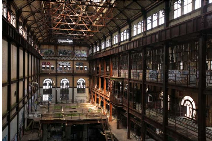
Figure 50: Interior of Turbine Hall Credit: Will Ellis
