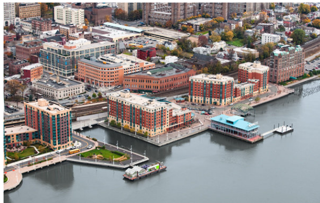
Figure 26: Aerial of Downtown Yonkers Waterfront Credit: Perkins Eastman
