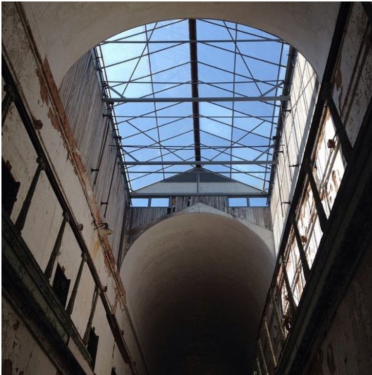
Figure 5. Cellblock seven skylight. Photo by the author, August 2014.
