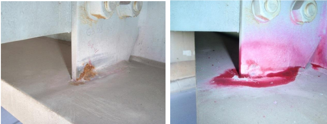
(a) Girder 3 Bay 2 Diaphragm 3
