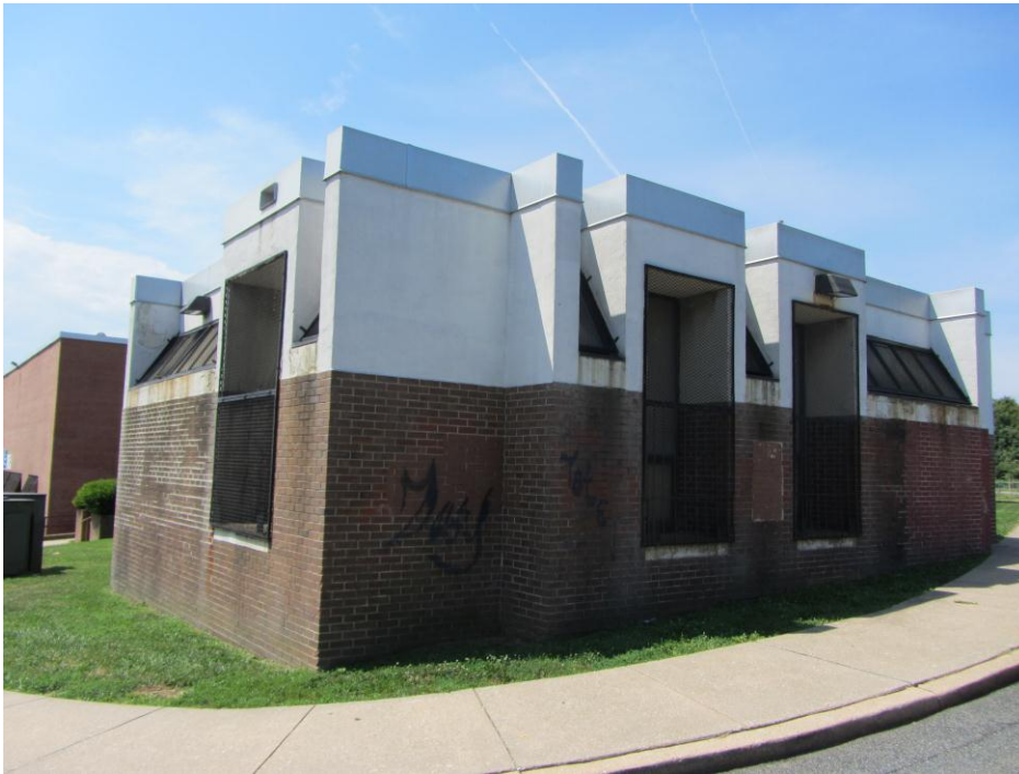
Figure 2.9 - Bentalou Recreation Center – Side (Photo by Author)
