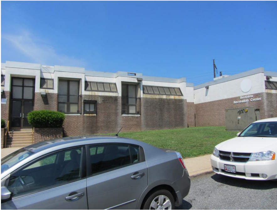
Figure 2.8 - Bentalou Recreation Center – Front (Photo by Author)
