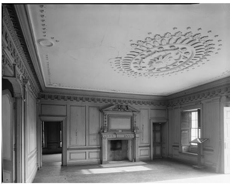
FIGURE E: Drayton Hall Ballroom, Historical Survey of American Buildings, Library of Congress.
