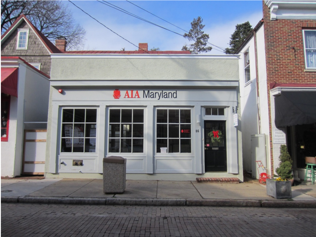
Figure 18: Southeast elevation of 86 Maryland Avenue's commercial addition.
