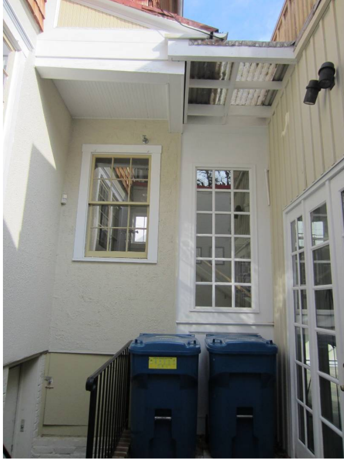
Figure 19: Southwest elevation of 86 Maryland Avenue's small addition and the stair connector.
