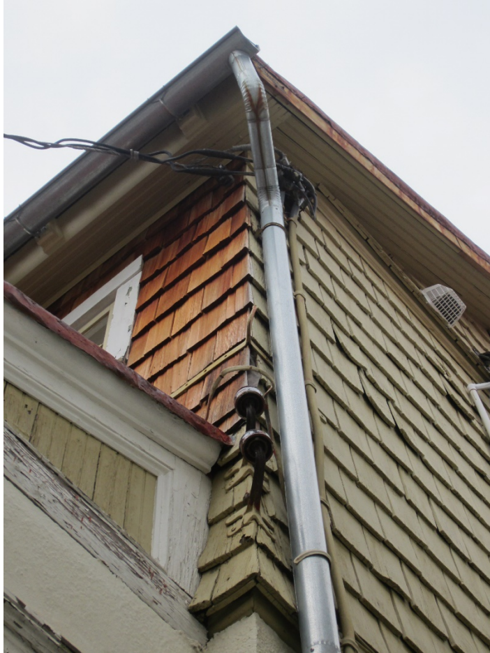
Figure 17: Eastern corner of 86 Maryland Avenue showing the painted and unpainted shingles.
