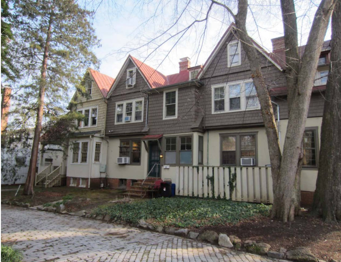
Figure 15: Northwest elevation of 1, 2 and 3 Randall Court.
