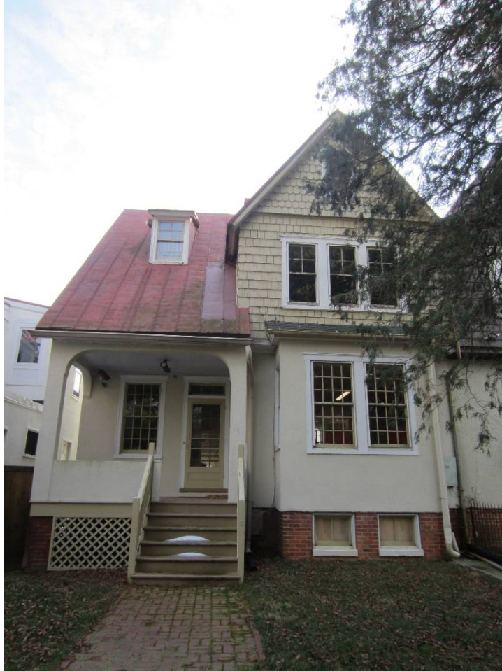
Figure 16: Northwest elevation of 86 Maryland Avenue / 3 Randall Court.
