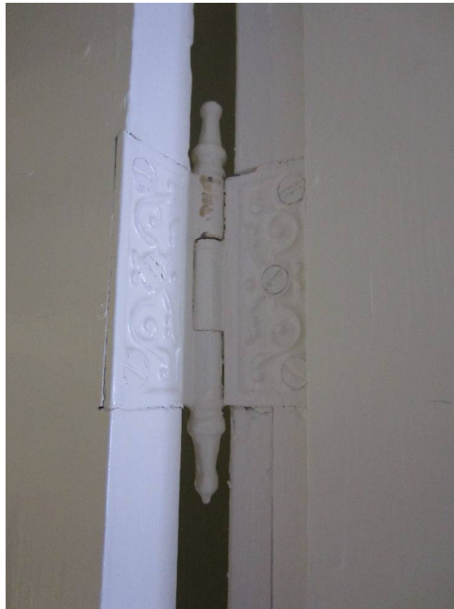
Figure 22: Historic door hinges on a door on the third floor.
