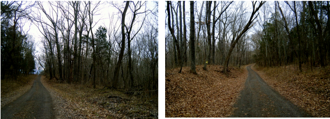
Figure 24: Views down Rogues Road when coming from Germantown Road. Road is noticeably sunken and not paved (photographed by author).
