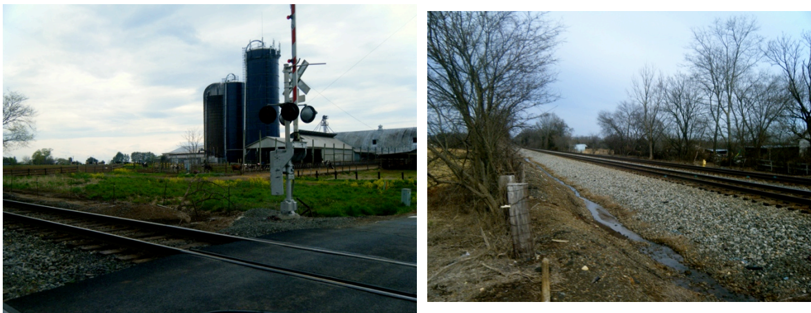
Figure 26: View of Norfolk Southern Rail Road from Road. From this image one can see the proximity of railroad to the dairy (photographed by author).
