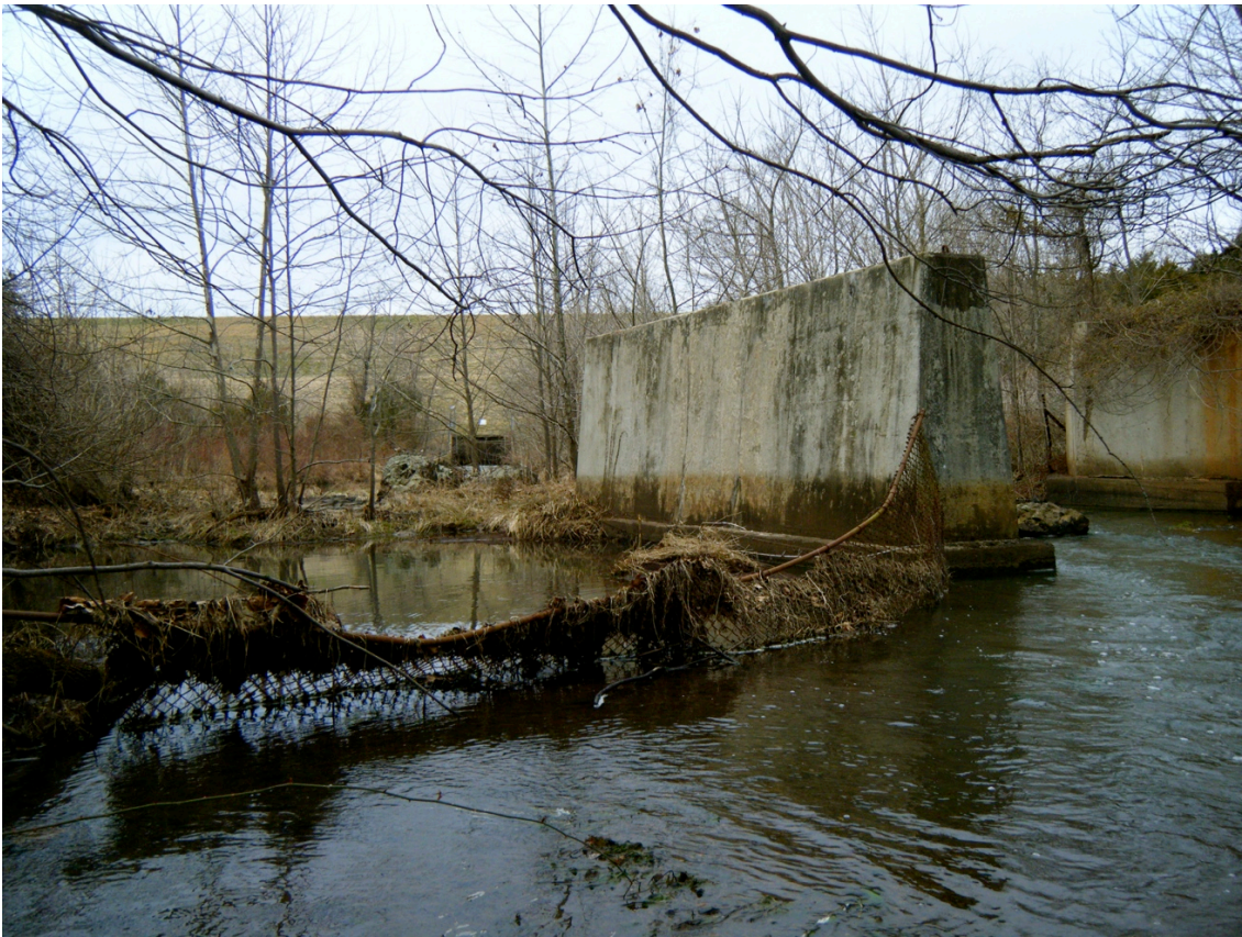
Figure 20: View of back of dam from dead end of Rogues Road with modern bridge over Licking Run that was destroyed most likely when the dam was built (photographed by author).
