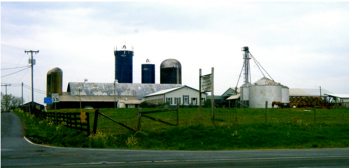
Figure 33: Closer up on the dairy portion of the Cow-N-Corn complex. This is a family farm which has existed since the 1930's and was specifically chosen because the property is cut through by the railroad. They have been dairying since 1954 and still focus on that today as well as agri-tourism ( http://www.cows-n-corn.com/ , photographed by author).
