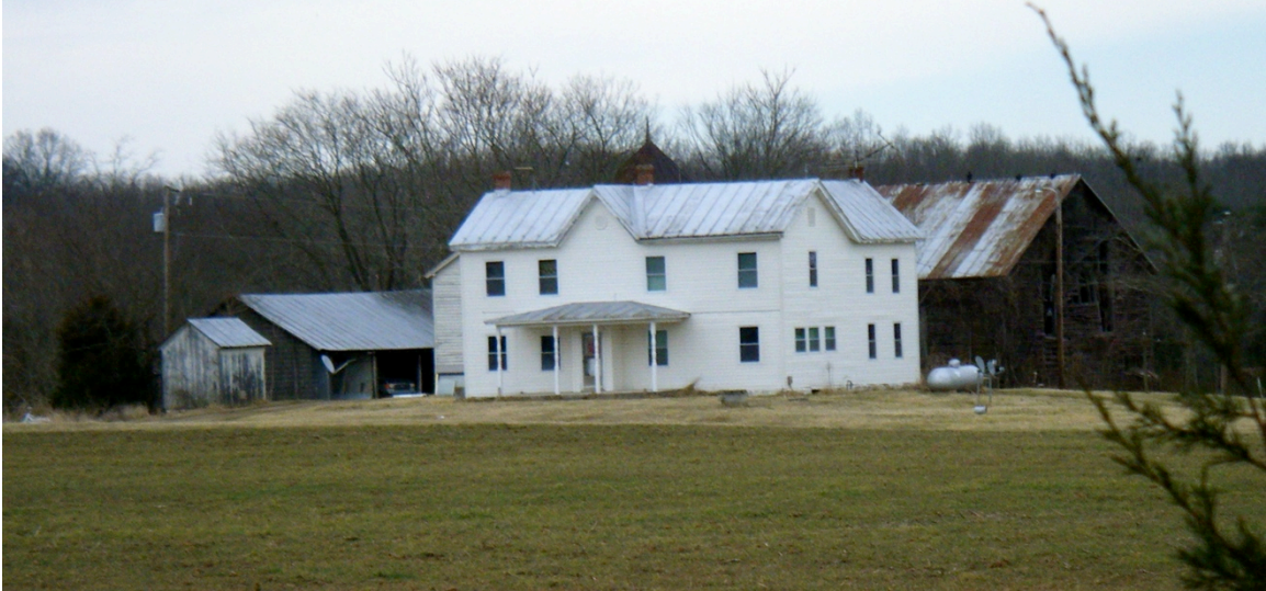
Figure 30: The Martin House with various outbuildings seen behind (photograph taken by author).
