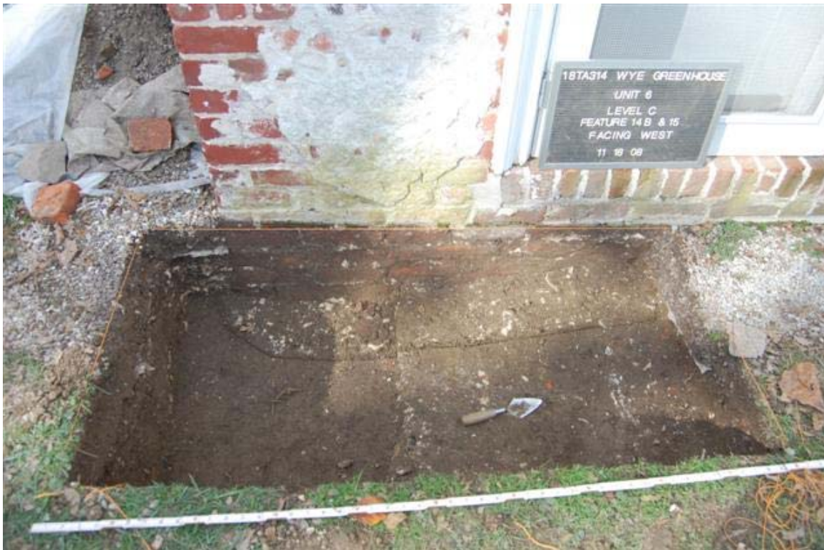
Figure 5.31– Unit 6 Feature 15 – This is the builders' trench for the east wall of the Greenhouse. The trench exposed a seven layer brick foundation. Photograph by John Blair.
