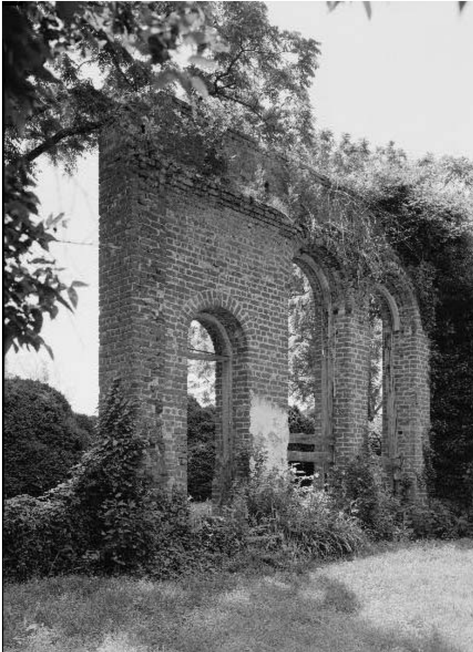
Figure 3.11 – The Ruins of the Greenhouse at Mount Airy, Richmond County, Virginia. The wall of the south façade is all that survives from what was once the crowning jewel on this impressive estate. Photo retrieved from HABS database.
