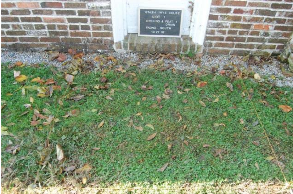
Figure 5.1 – Unit 1 Level A and Modern Drain (Feature 1) – This is the existing condition of Unit 1 prior to excavation. Photo by Matthew Cochran
