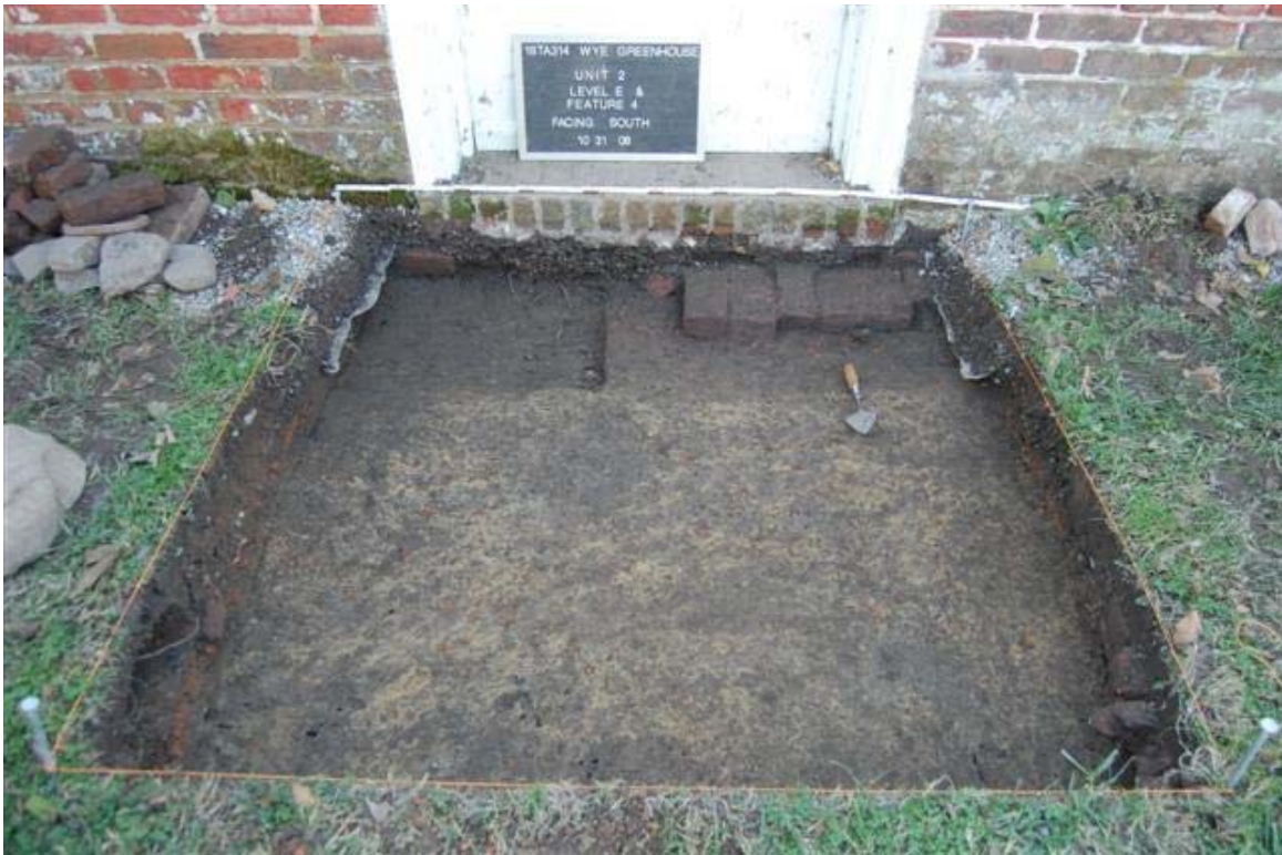
Figure 5.8 – Unit 2 Drip Line (Feature 4) – The Builder’s Trench revealed a dry-laid foundation supporting the living quarter behind the main block of the greenhouse. The clay subsoil showed “pockets” or small voids, most likely due to rodent and root disturbance. Photo by Stephanie Duensing
