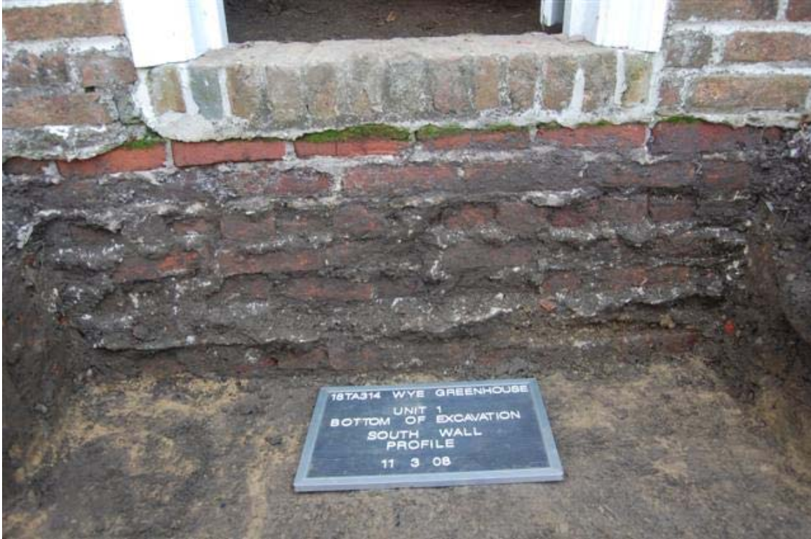
Figure 5.3 – Unit 1 Foundation – This is a photograph that shows the mortar being compressed between the bricks so that that mortar has come out the front of the bricks and has set on the face of them. Photograph by John Blair.
