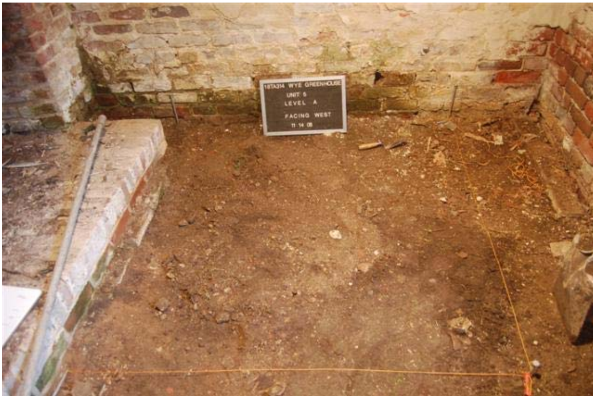
Figure 5.27 – Unit 5 Level A1 – This is the existing condition of Unit 5 prior to excavation. Photo by Matthew David Cochran
