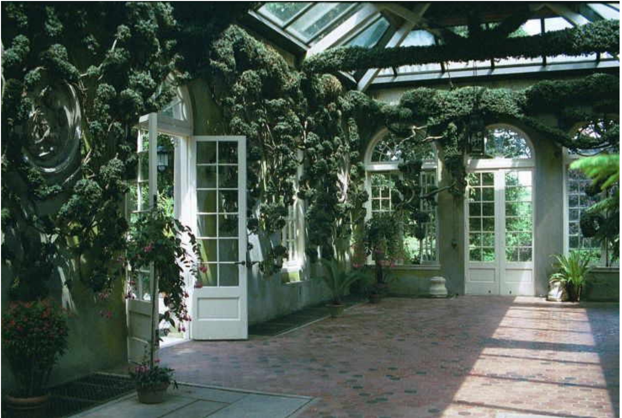
Figure 3.14 – The Greenhouse at Dumbarton Oaks in Washington, D.C. – Pictured here can be seen the vastly different utilization of glass and window features. This new experimentation with light and glass was a mile marker in the stylistic advancements and benefits of better and more scientific methods of construction. Photo retrieved from www.gardentraveler.com
