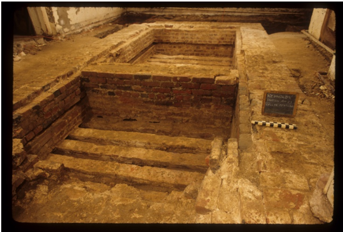
Figure 4.57: Brick storage feature in basement, facing east.
