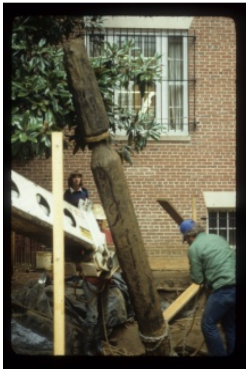
Figure 4.39: Crew using pulley system to remove water pipe from well.
