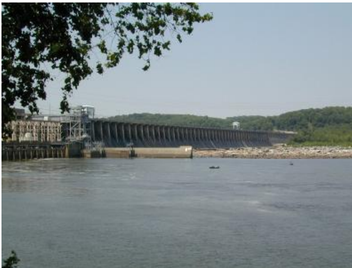
Figure 3.3 Photo of the Conowingo Dam in located Maryland. Photo taken from USGS.gov.
