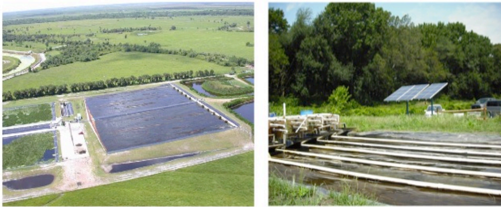
Figure 1.4 Different scale ATS systems. The system on the left shows an industrial-scaled ATS at 1 hectare in Florida and able to process 10 million gallons per day (HydroMentia Inc., n.d.). Picture courtesy of HydroMentia, Inc. The system on the right is a solar-based system constructed on a farm near Bridgetown, Maryland with dimensions of 6 meters wide and 50 meters long.
