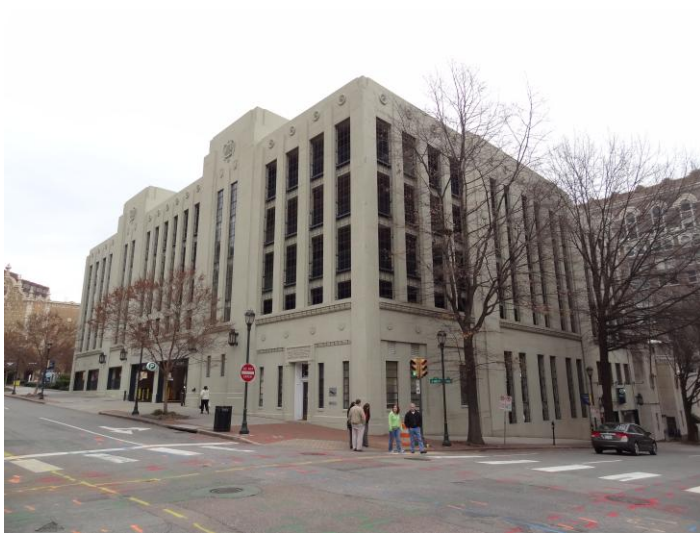
Figure 53. Existing parking garage on southwest corner of site
