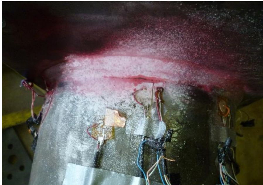
Figure 4.7. Crack at the weld toe of test specimen (dark red line identified with dye penetrant)
