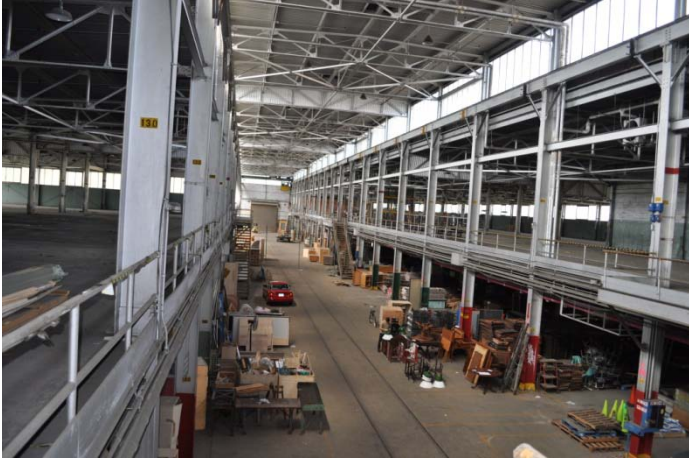
Figure 36. Double-height central space (Source: Author)
