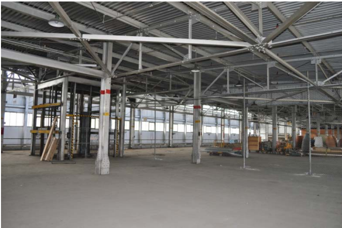
Figure 37. Second floor with elevator shaft (Source: Author)
