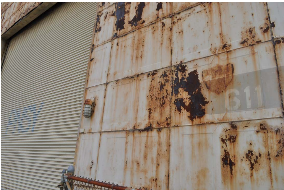
Figure 32. Exterior steel cladding (Source: Author)
