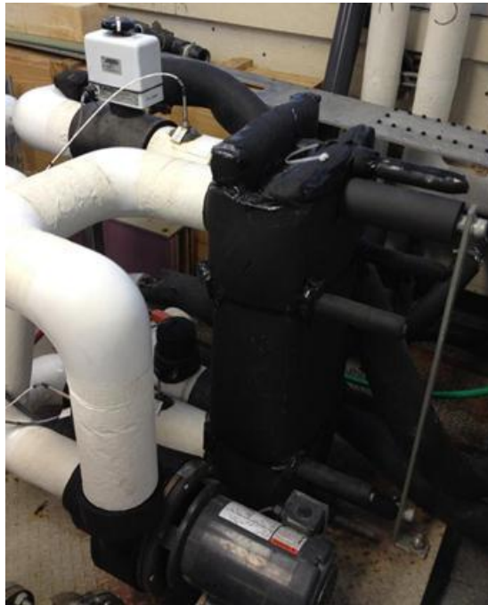
Figure 24: Water-to-water/glycol PHE
