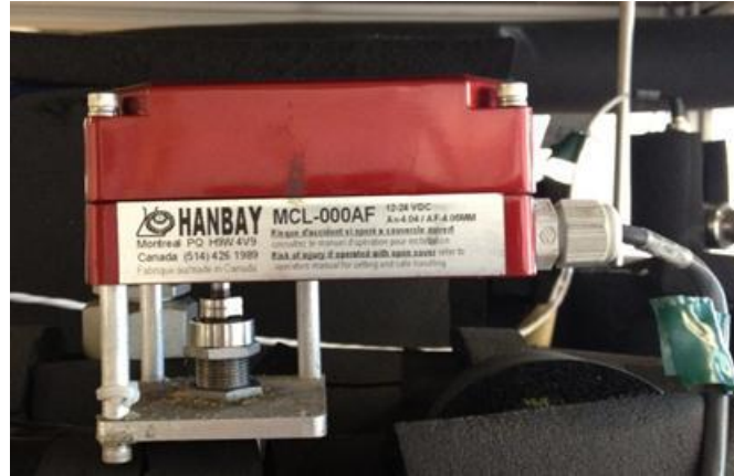
Figure 21: EXV and its actuator
