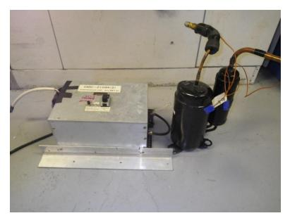
Figure 64: The variable speed compressor and its inverter
