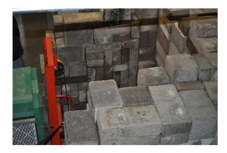
Figure 8. Concrete walls built for shielding of east wall of reactor building.
