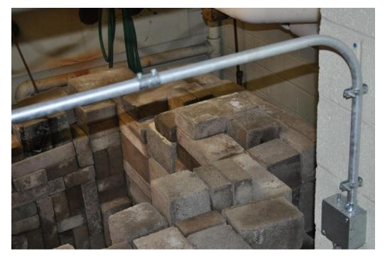
Figure 8-5: U-shaped concrete walls built along east wall of reactor building. The walls are 24 inches thick and 7 feet high.
