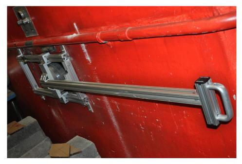
Figure 8-3: The shutter system installed in front of the East Beam Port. The shutter is attached to the concrete of the reactor and is able to provide a shutter for either the beam port or the through tube.
