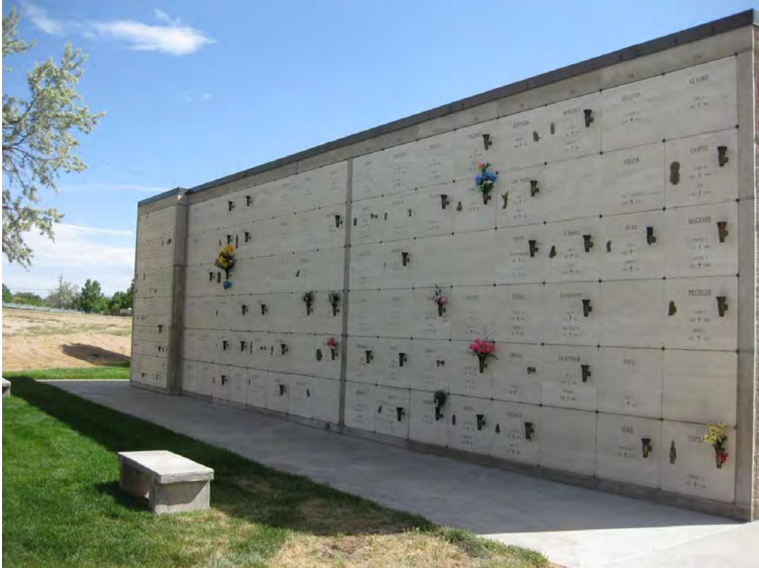
Figure 68-typical mausoleum exterior (Source: author)
