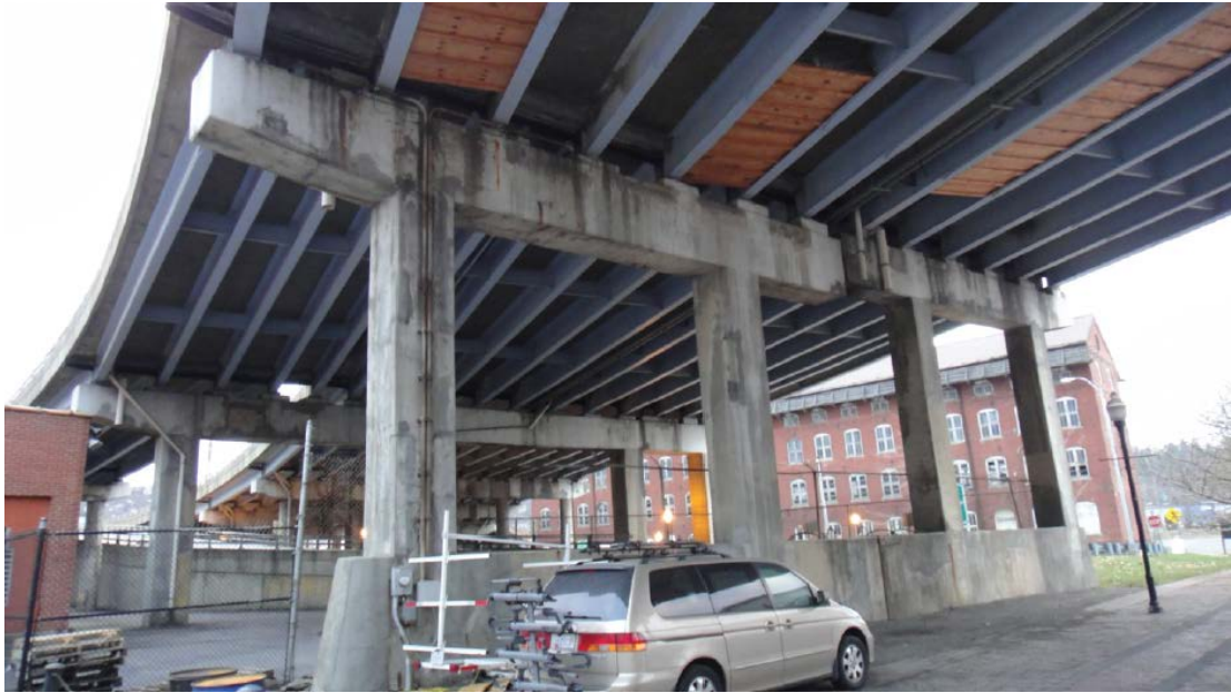
Figure 25 – Under-Highway Condition (Source: Author)
