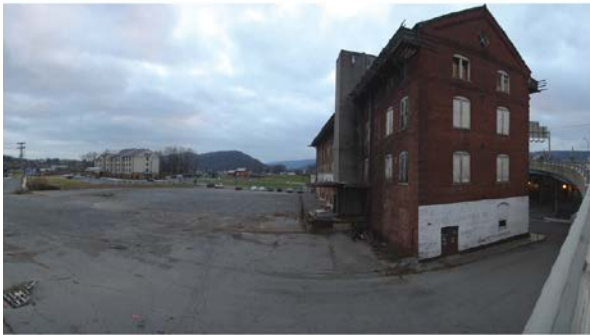
Figure 14 - Historic Footer Building Location and Situation
