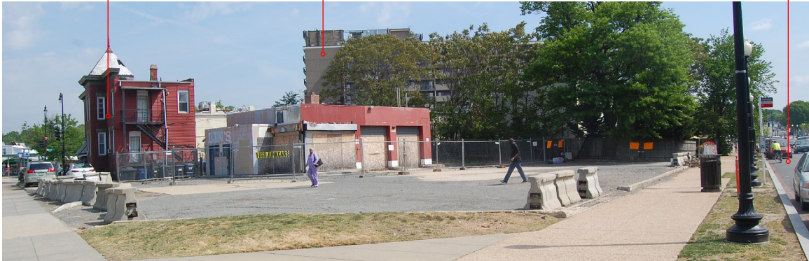
Figure 60 Site Conditions - 1400 Maryland Ave. NE [Sickle]
