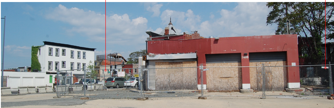
Figure 61 Site Conditions - 1400 Maryland Ave. NE [Sickle]
