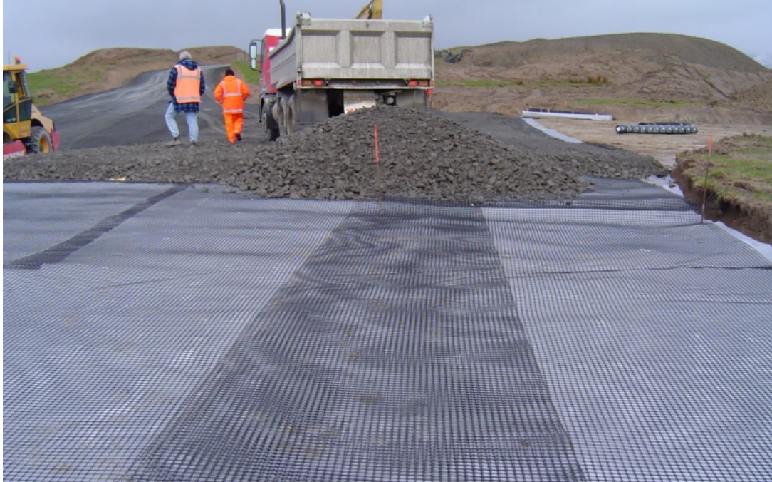
Figure 5.3- Construction site of project B – Road improvement project
