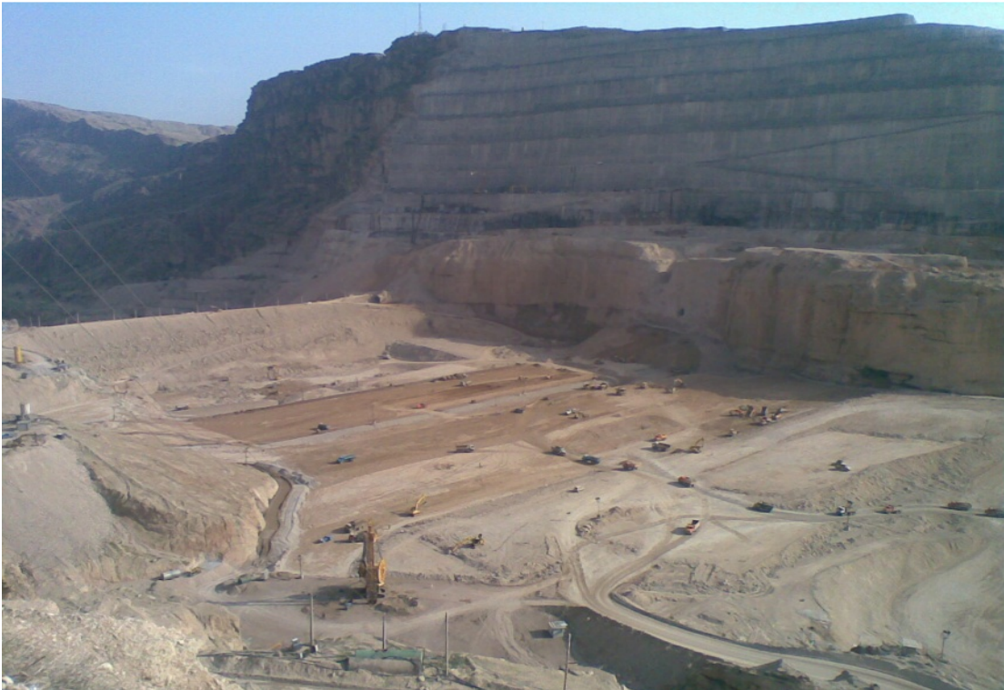
Figure 5.1- Construction site of project A – Reservoir earth dam project
