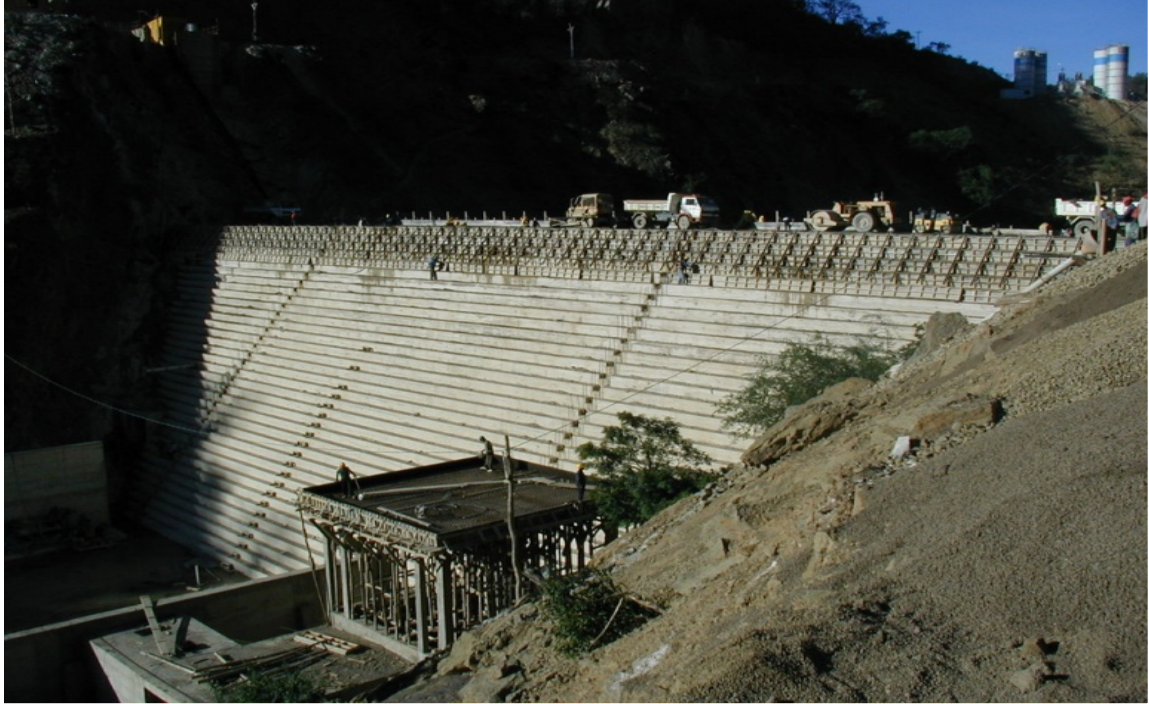
Figure 5.7- Construction site of project D – Reservoir concrete dam project
