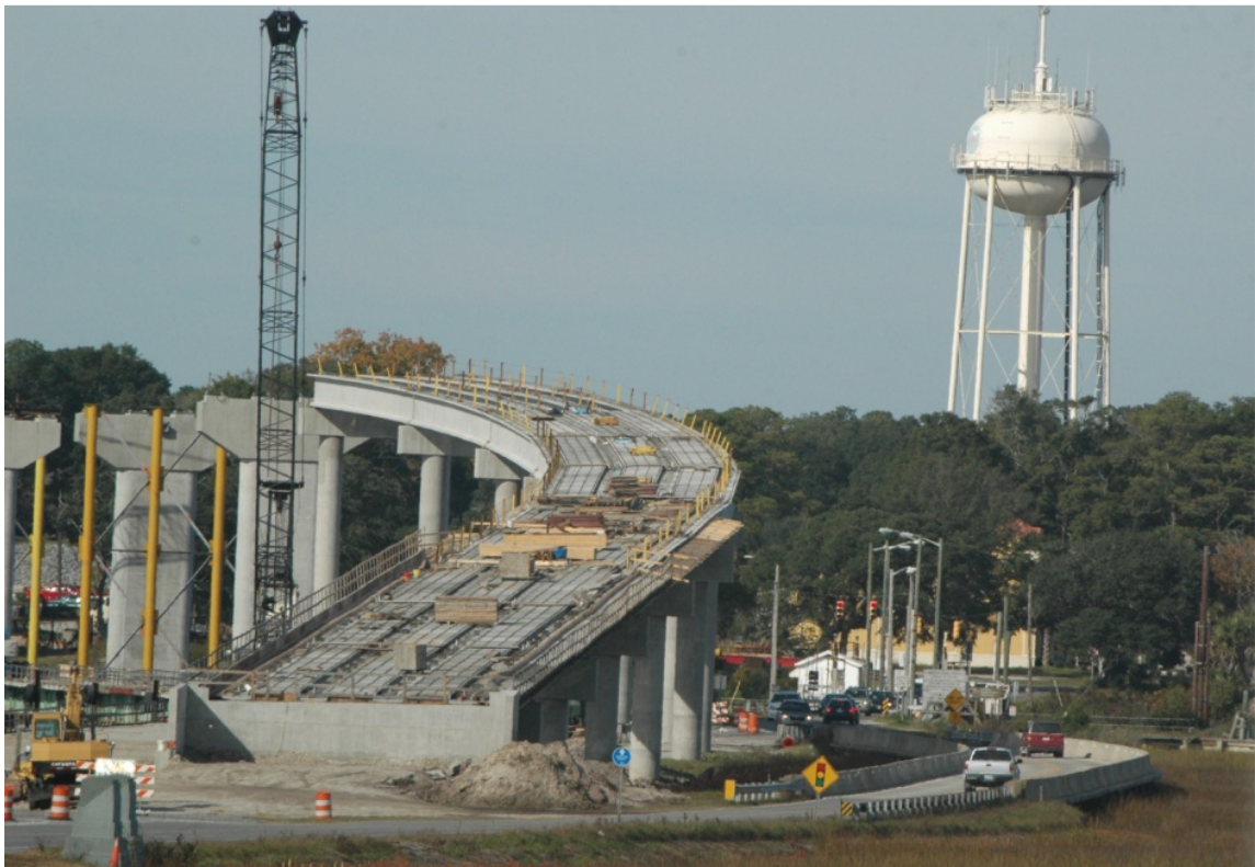
Figure 5.5- Construction site of project C – Road construction project
