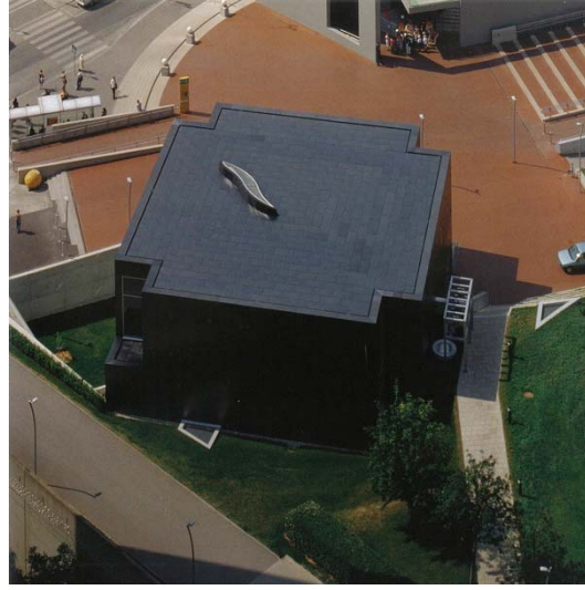
Fig. 01, The ascetic interior offers few clues of the outside world. Fig. 02, The black steel cube stands out sharply in the urban context.
