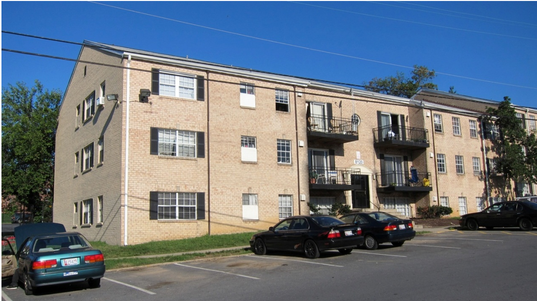
Fig. 30, Typical garden apartment building in Langley Park.
