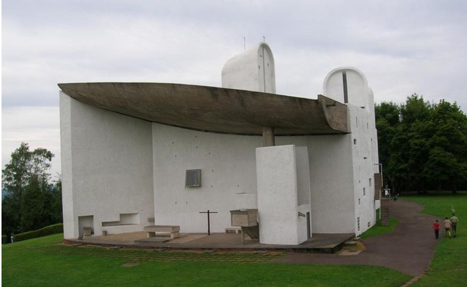
Fig. 09, The east porch is meant for outdoor public mass.
