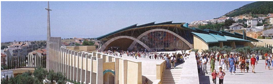
Fig. 07, A pilgrimage church, the plaza is meant as a public gathering place.
