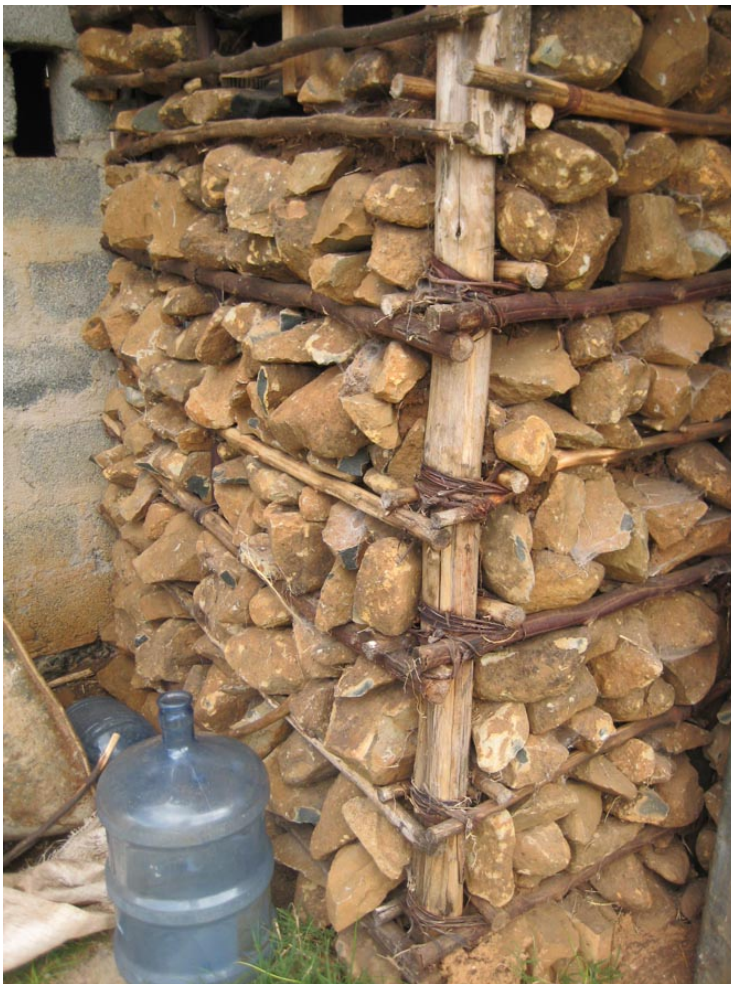
Figure 2.2. Construction with readily available, local materials. Image by Author.
