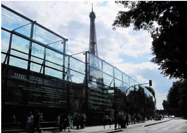
Figure 21_The glazed palisade of the Musée du Quai Branly creates a visual complexity of reflection, and informs by the application of graphic text (source: author)
