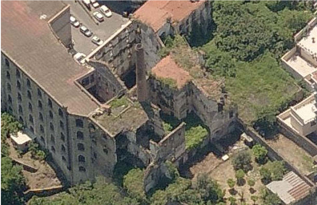
Figure 6-2-13. Building shell. Bird's eye view looking south.
