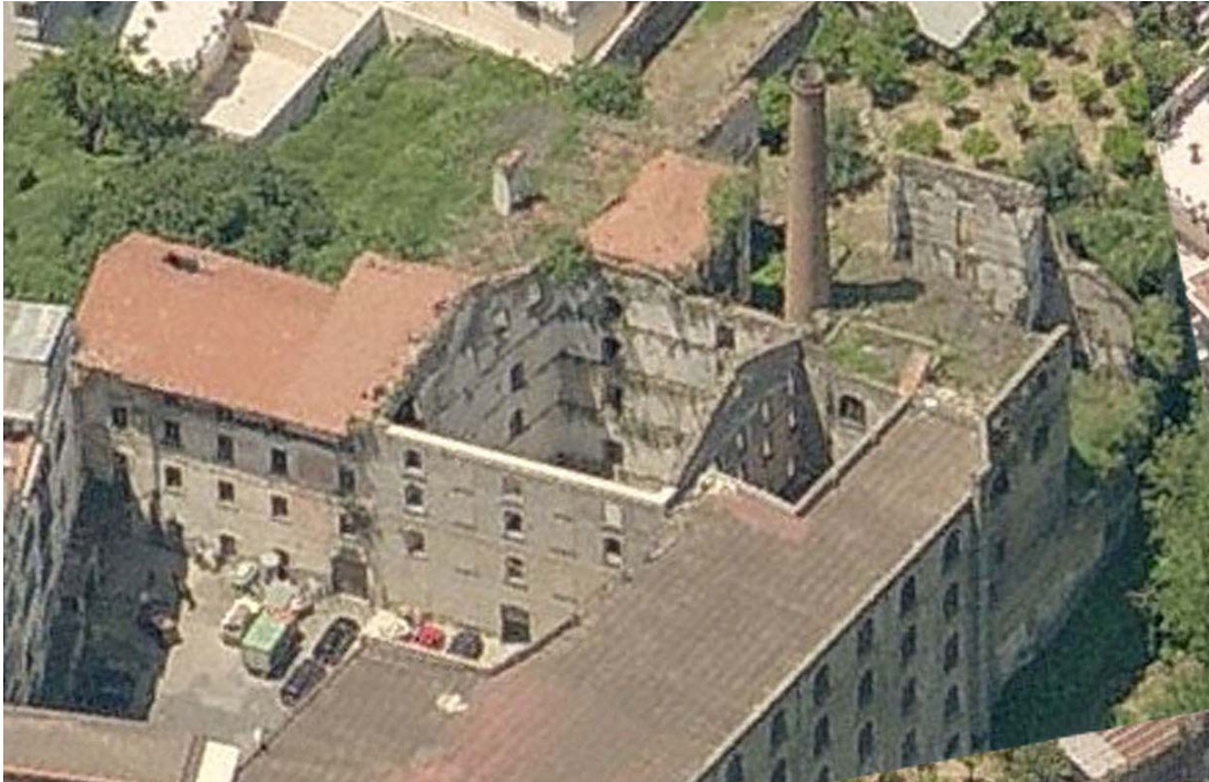
Figure 6-2-15. Building shell. Bird's eye view looking west.
