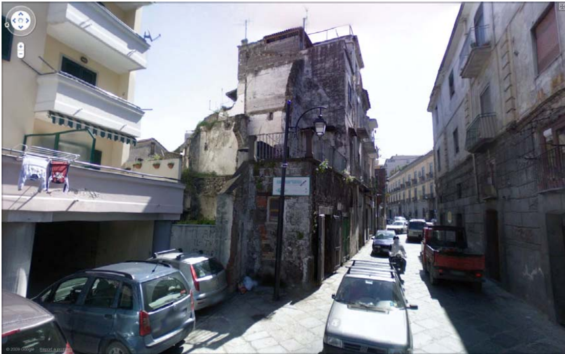
Figure 6-3-5. Looking southeast at the choke to Via Roma.
