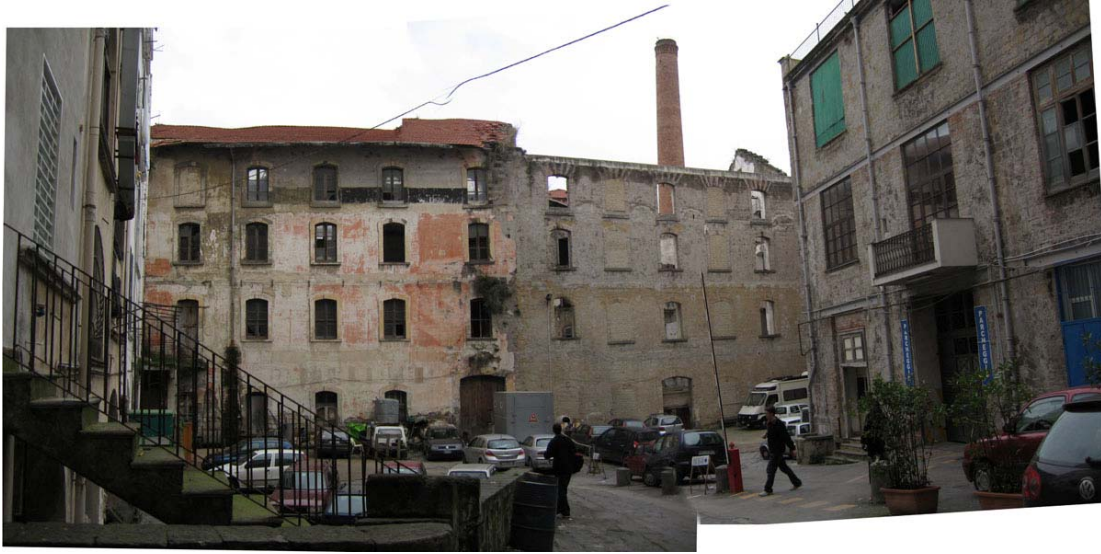
Figure 6-2-1. View of historic building shell from enclosed courtyard.
