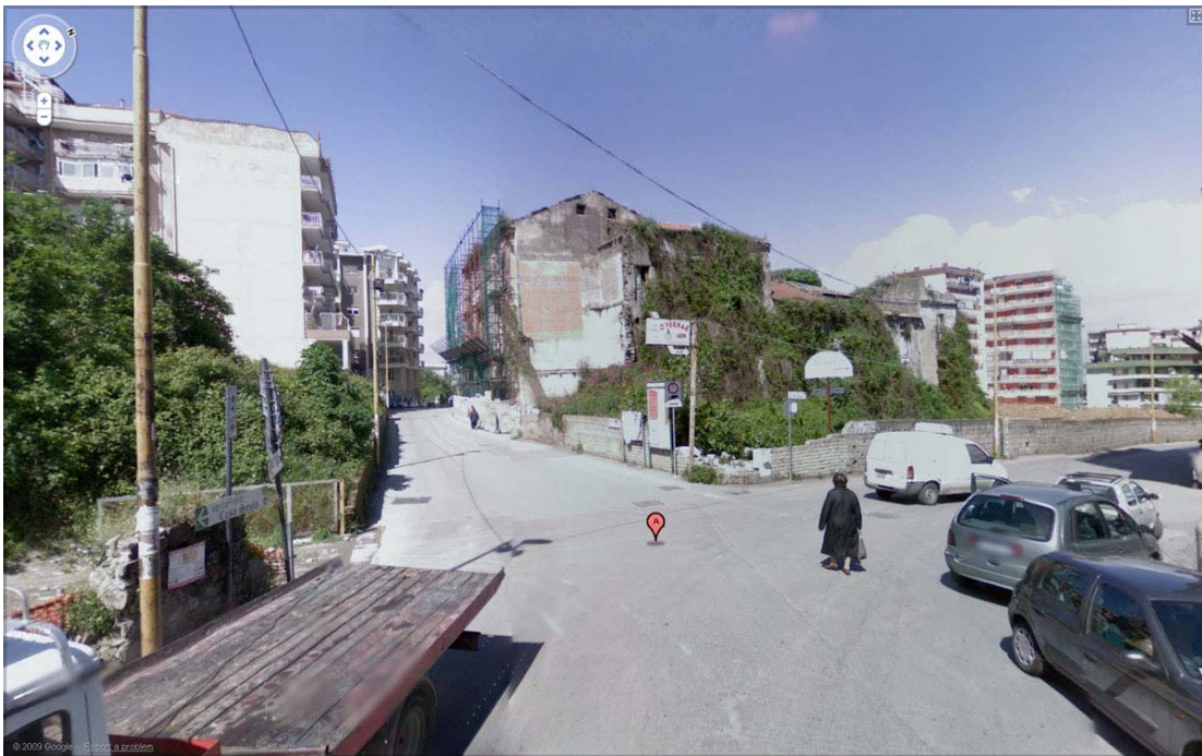
Figure 6-3-3. At Piazza Trivione, entry to Via Roma, looking northwest.
