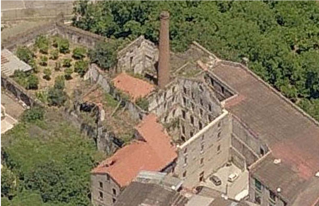
Figure 6-2-17. Building shell. Bird's eye view looking north.
