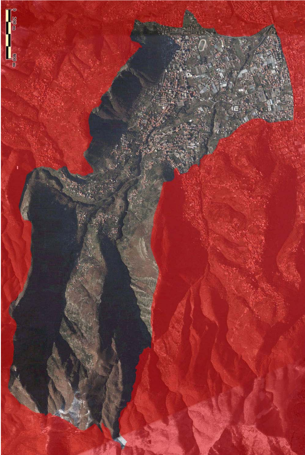
Figure 2-1-16. Aerial of the Gragnano Commune.
