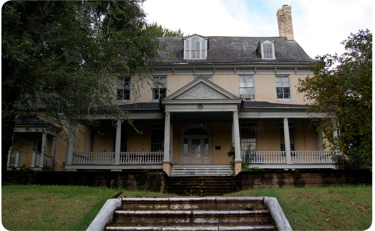
Bostwick Main House, looking east, Fall 2011.
