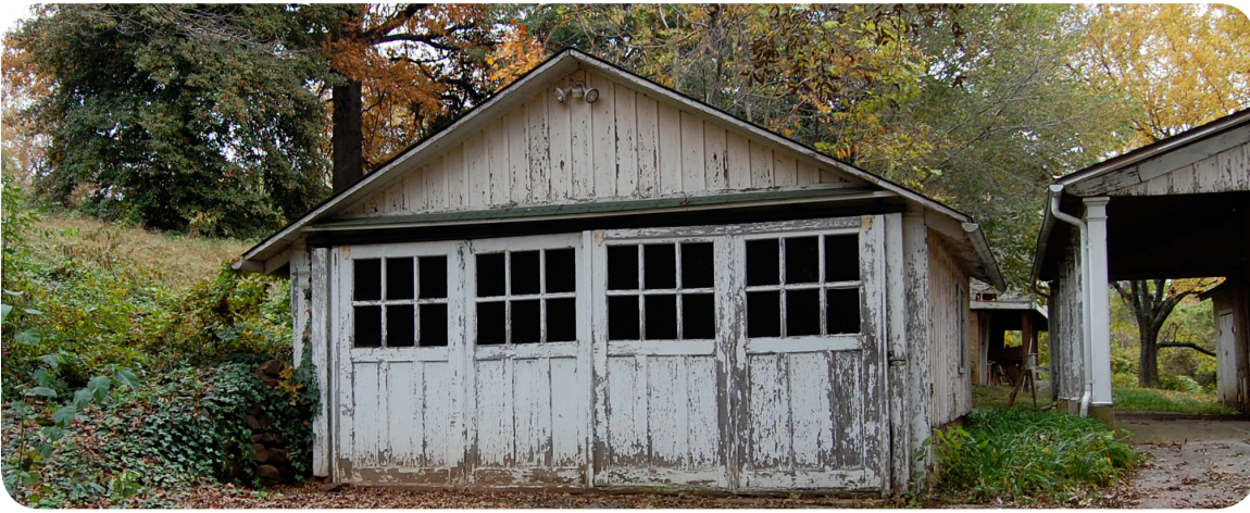
Garage, looking south, Fall 2011.
