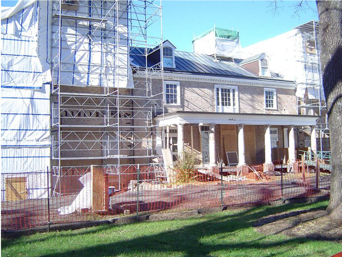
Figure 2.6 Montpelier during the restoration (photo from Wikicommons).
