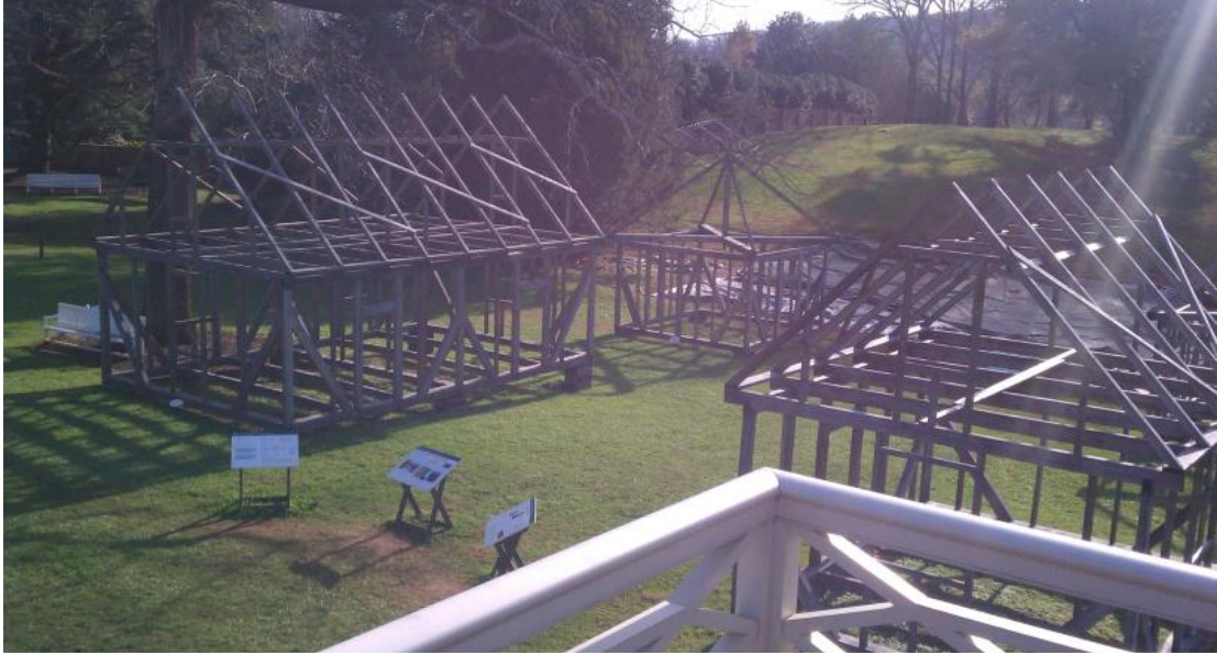
Figure 1.2. Reconstructed frames of slave quarters at Montpelier, as of early 2012 (photo by author).
