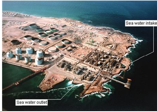
Figure 42: Das Island seawater intake and outlet [90]
