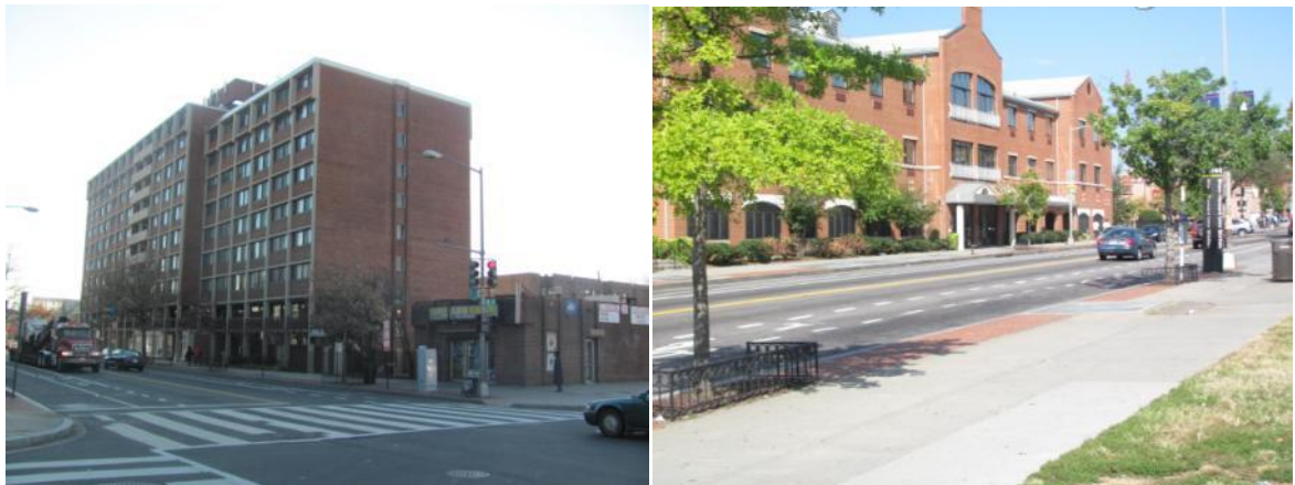
Figure 85: Adjacent Parcels. Conflicting Mix of Scale and Street Use
