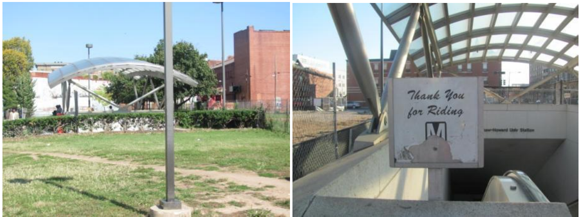
Figure 78: Existing Shaw Metro Canopy and Escalator Entrance
