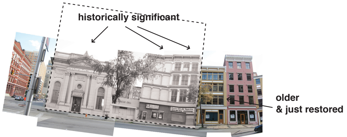
Figure 31_ Historical context images. cast iron fronts are to be restored in the architectural proposal, while the interior masonry bearing walls are to be torn down in order to insert the housing tower. retail use at the ground floor will be maintained here. the bank building will be restored to its original single volume space and a new skylight will be added.
