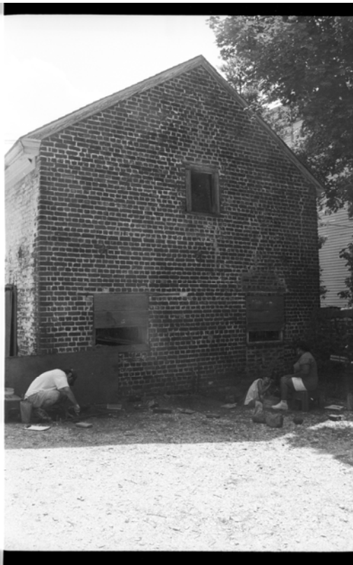
Figure 15: Photograph of Stables, Northeast Wall (Photo Courtesy of Brandon Grodnitzky.)
