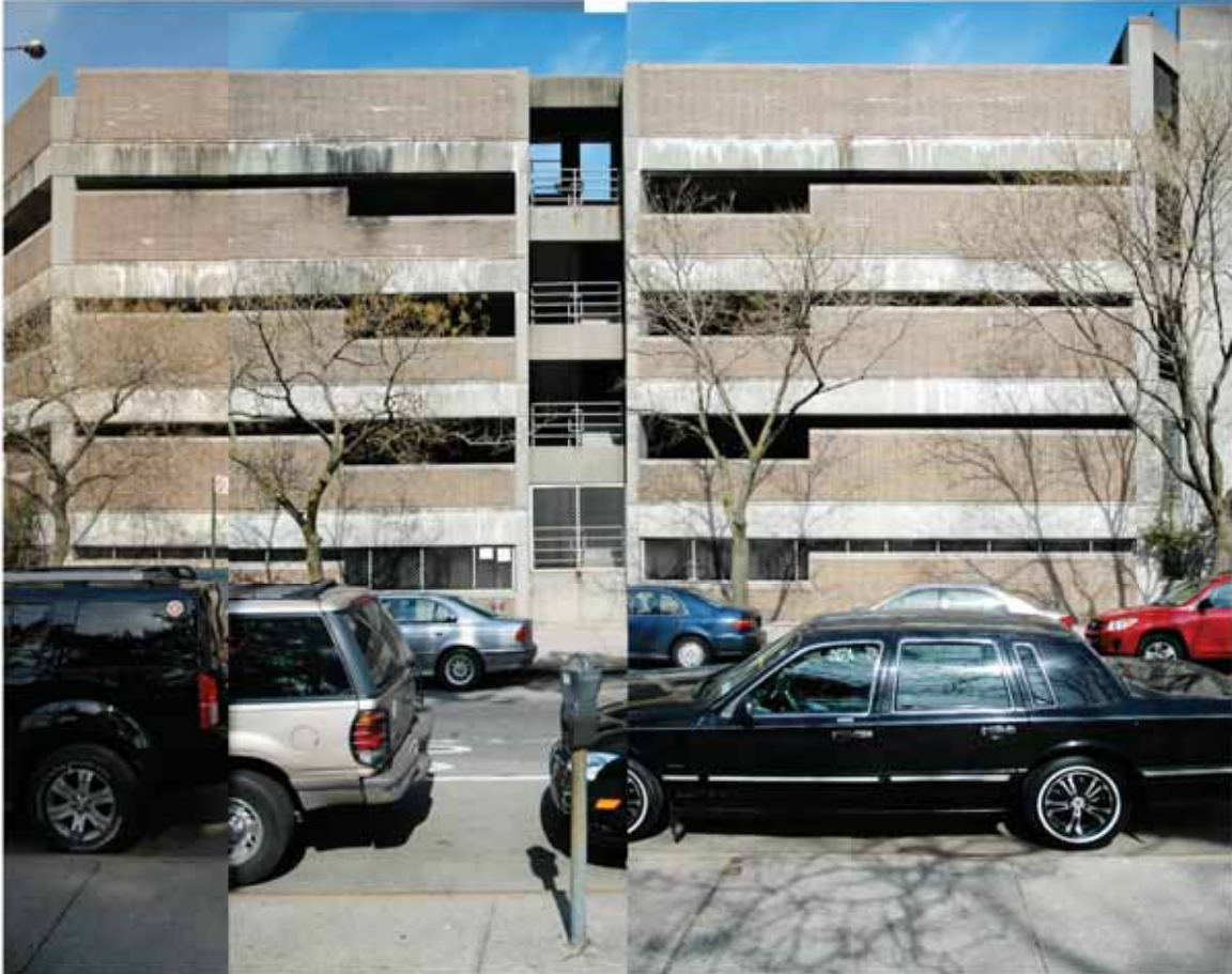
Figure 20 - Photographic elevation - Existing parking garage occupying Southwest corner of the former hospital site. Parking garage occupies significant corner facing Rufus King Park to the South.
