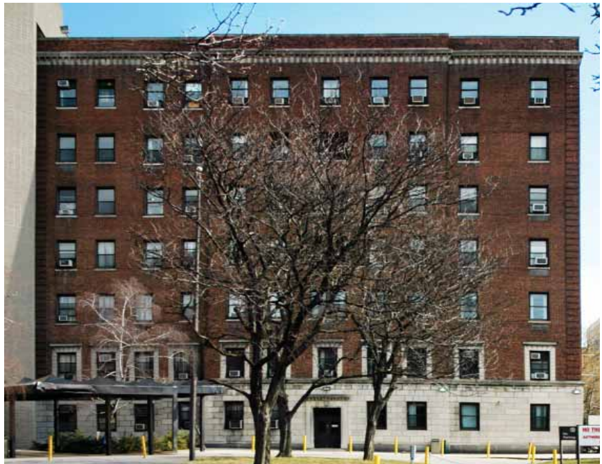
Figure 10 - Photographic Elevation - West facade of Existing Hospital wing, constructed c. 1926
