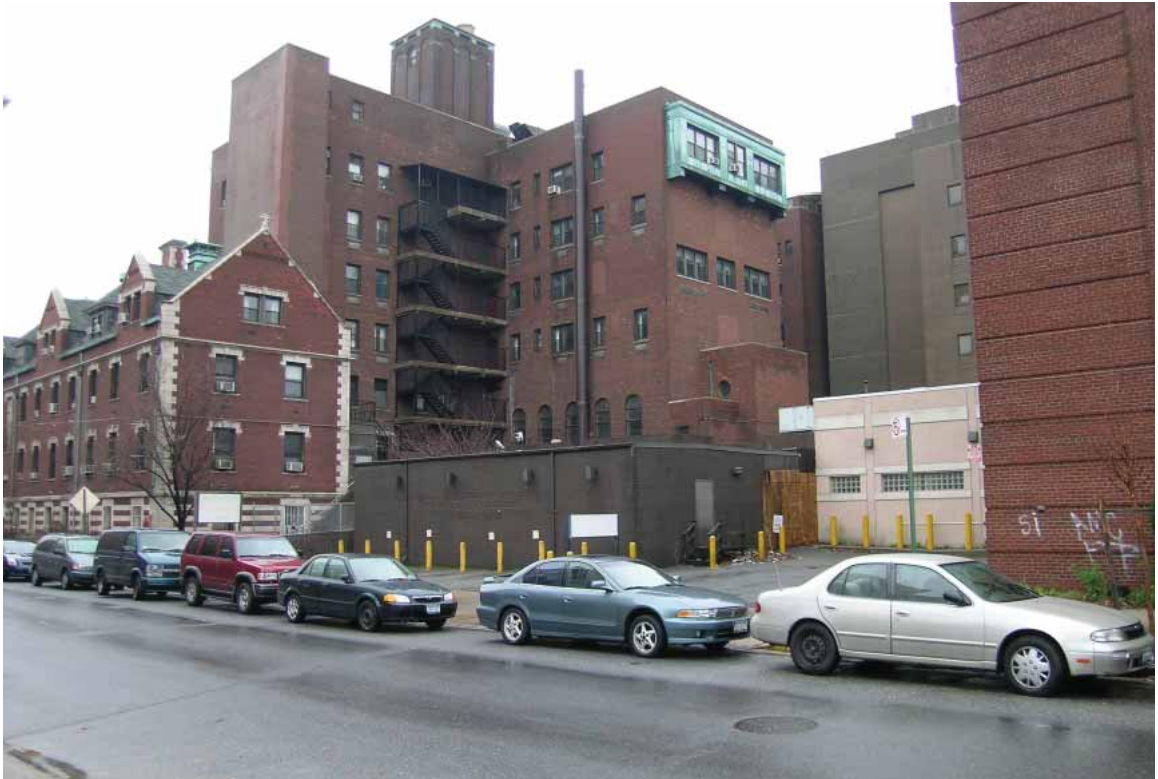
Figure 13 - View into site revealing various periods of construction
