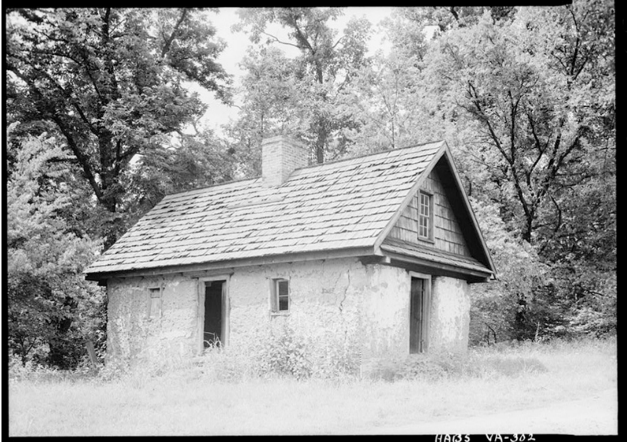
Figure 15. A rammed earth building at Bremo Recess, Brunswick County, Virginia (photograph from the Library of Congress, Prints and Photographs Division, Historic American Buildings Survey ).
