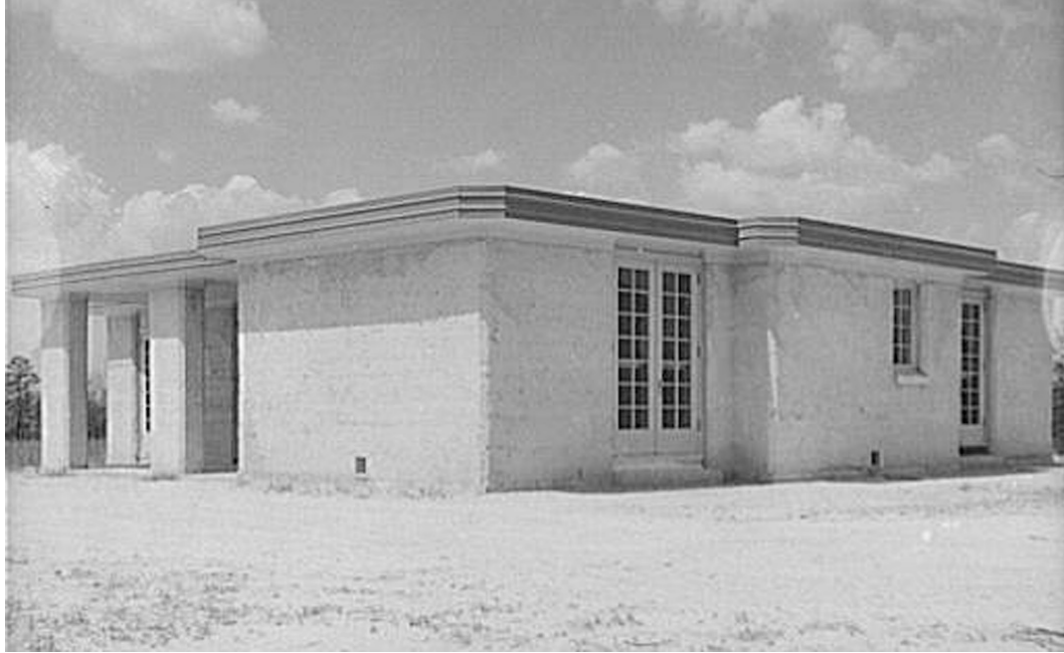
Figure 23. Side view of one of Gardendale's rammed earth homes, shortly after completion.
