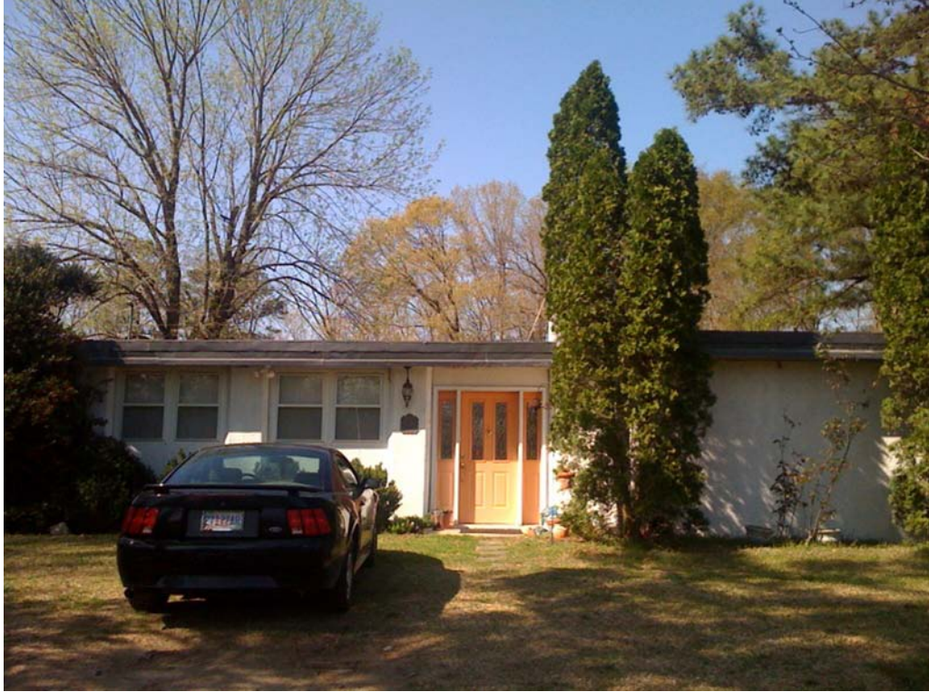
Figure 7. Façade of rammed earth house at 5350 Rosemary Road.
