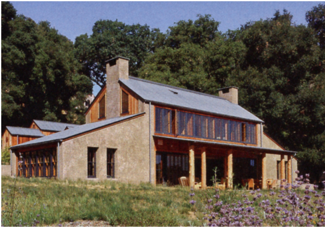
Figure 36. The Kavner house in northern California, built of rammed earth using the modern PISE technique ( image courtesy of Matthew Millman Photography and Turnbull Griffin and Haesloop. Used with permission. )
