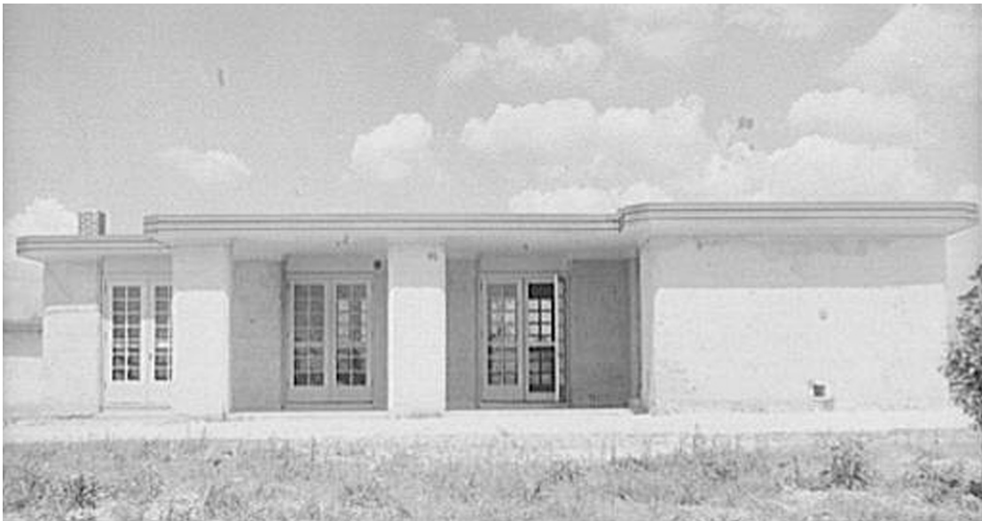
Figure 22. Rear view of one of Gardendale’s rammed earth homes, shortly after completion ( photographs from Library of Congress, Prints and Photographs Division ).
