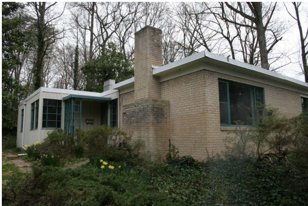
Figure 27. As the Parkbelt home with the most integrity, 7 Forest Way has recently attracted the attention of historic preservationists ( photographs by the author ).
