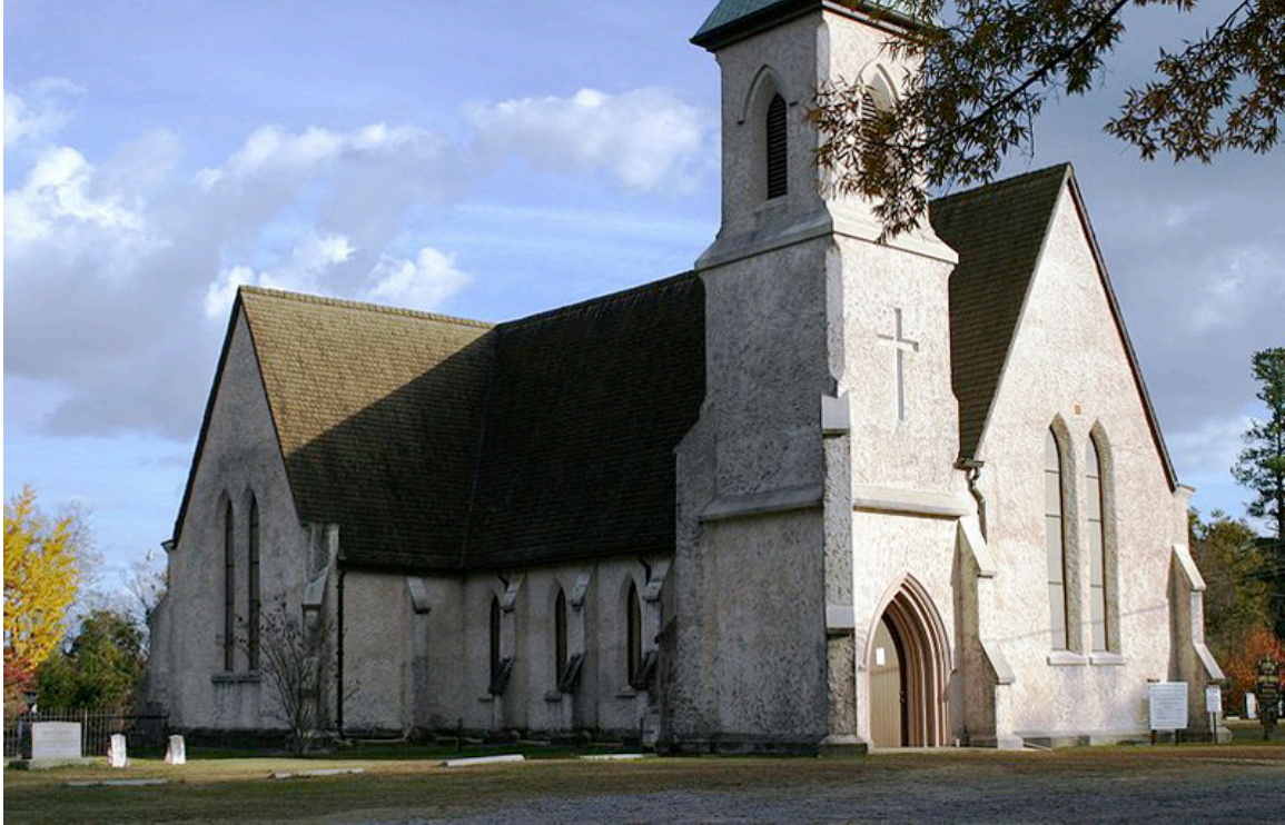
Figure 16. The Church of the Holy Cross in Stateburg, South Carolina, built of rammed earth, is listed in the National Register of Historic Places and is a National Historic Landmark (photograph courtesy of Wikipedia user Pollinator) .
