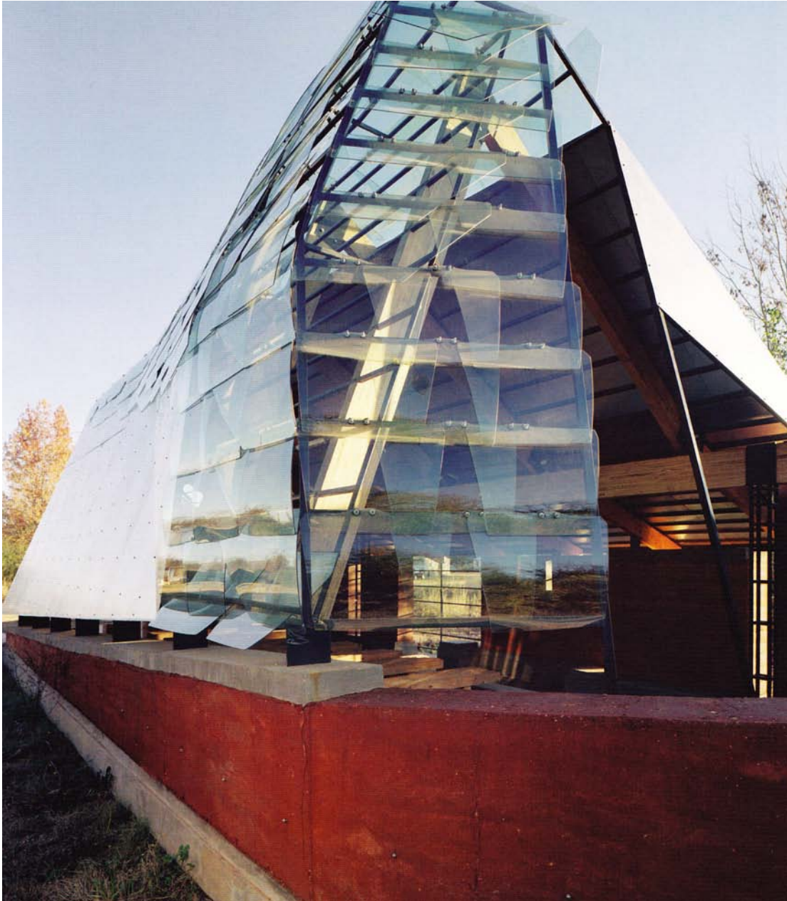
Figure 40. Mason's Bend Community Center, built by The Rural Studio out of unconventional materials, includes a rammed earth wall ( image from Earth Architecture by Ronald Rael, © Princeton Architectural Press. Used with permission. ).
