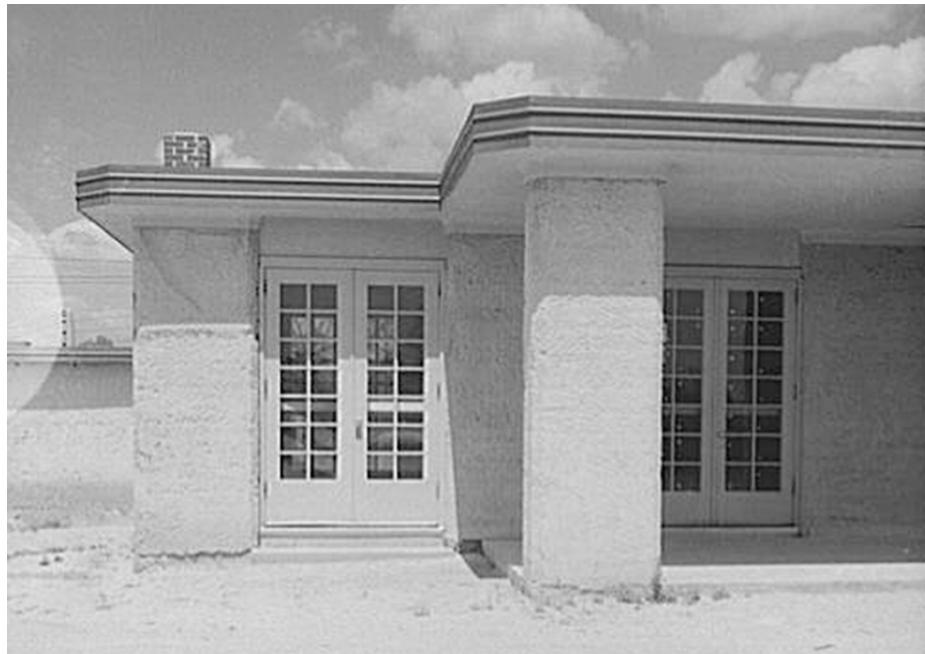
Figure 24. Gardendale's rammed earth homes used French doors to help with air circulation ( photographs from the Library of Congress, Prints and Photographs Division ).
