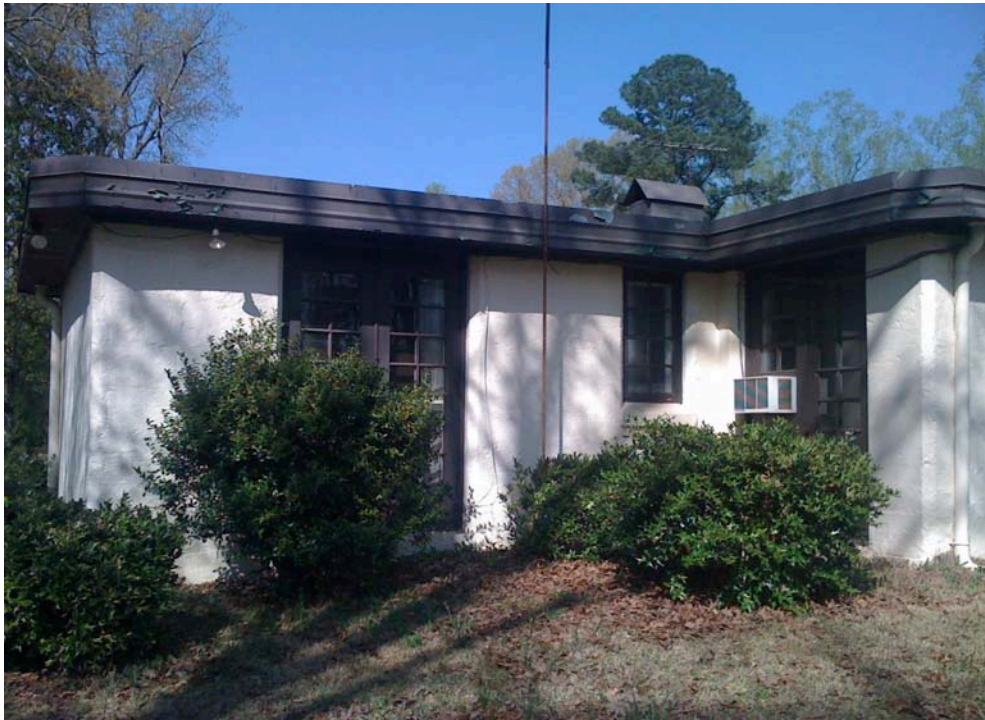
Figure 41. Gardendale’s rammed earth homes did not include a HVAC system; some residents have since installed such systems or window units.
