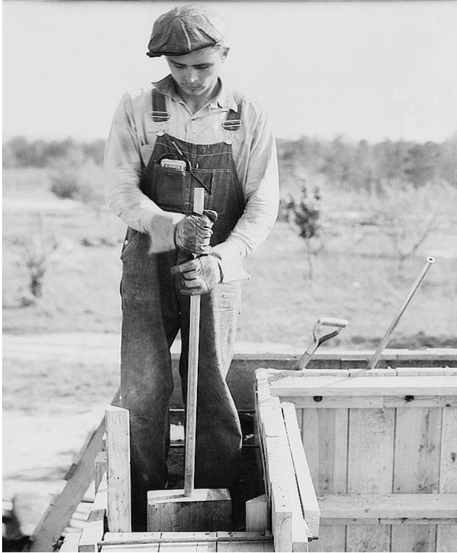
Figure 11. Workman tamping damp earth at Gardendale.
