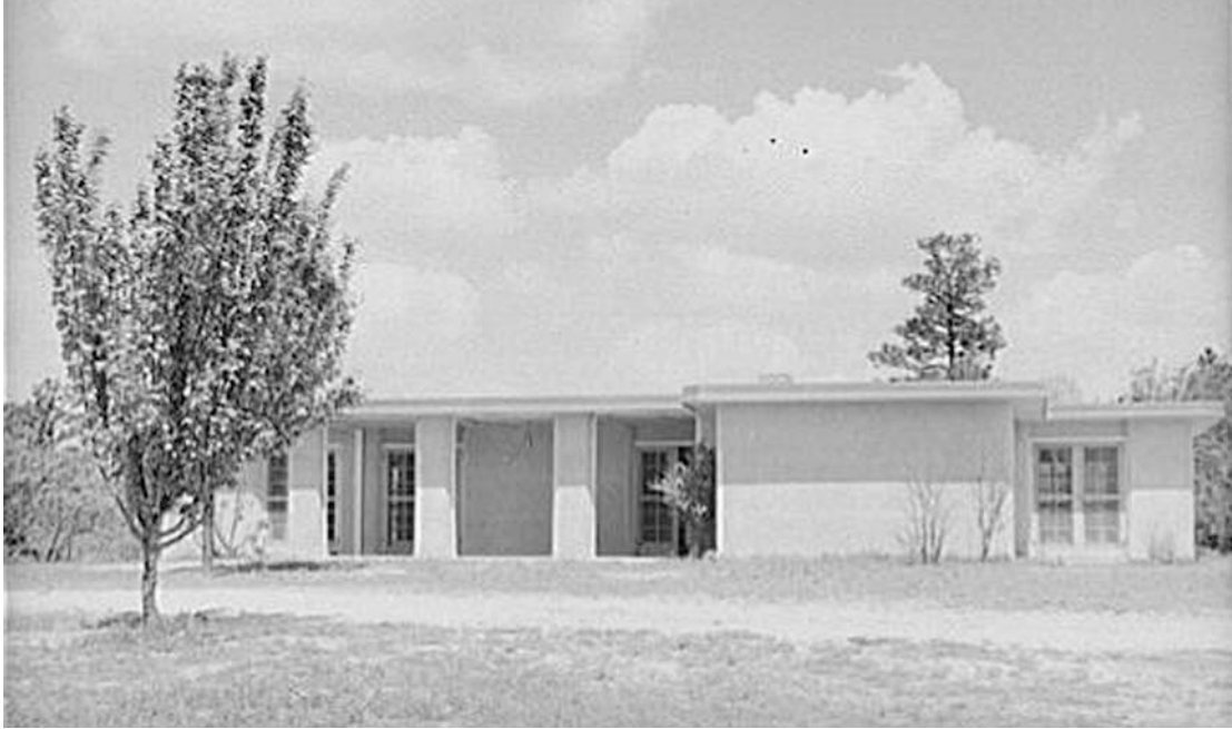
Figure 21. The façade of one of Gardendale’s rammed earth homes, shortly after completion.
