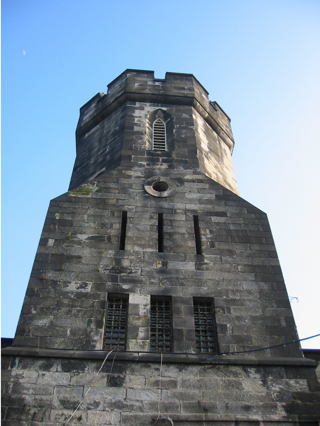
Figure 7: Front entrance of Eastern State Penitentiary. Photo courtesy of Steve Schwartzman, 2009.
