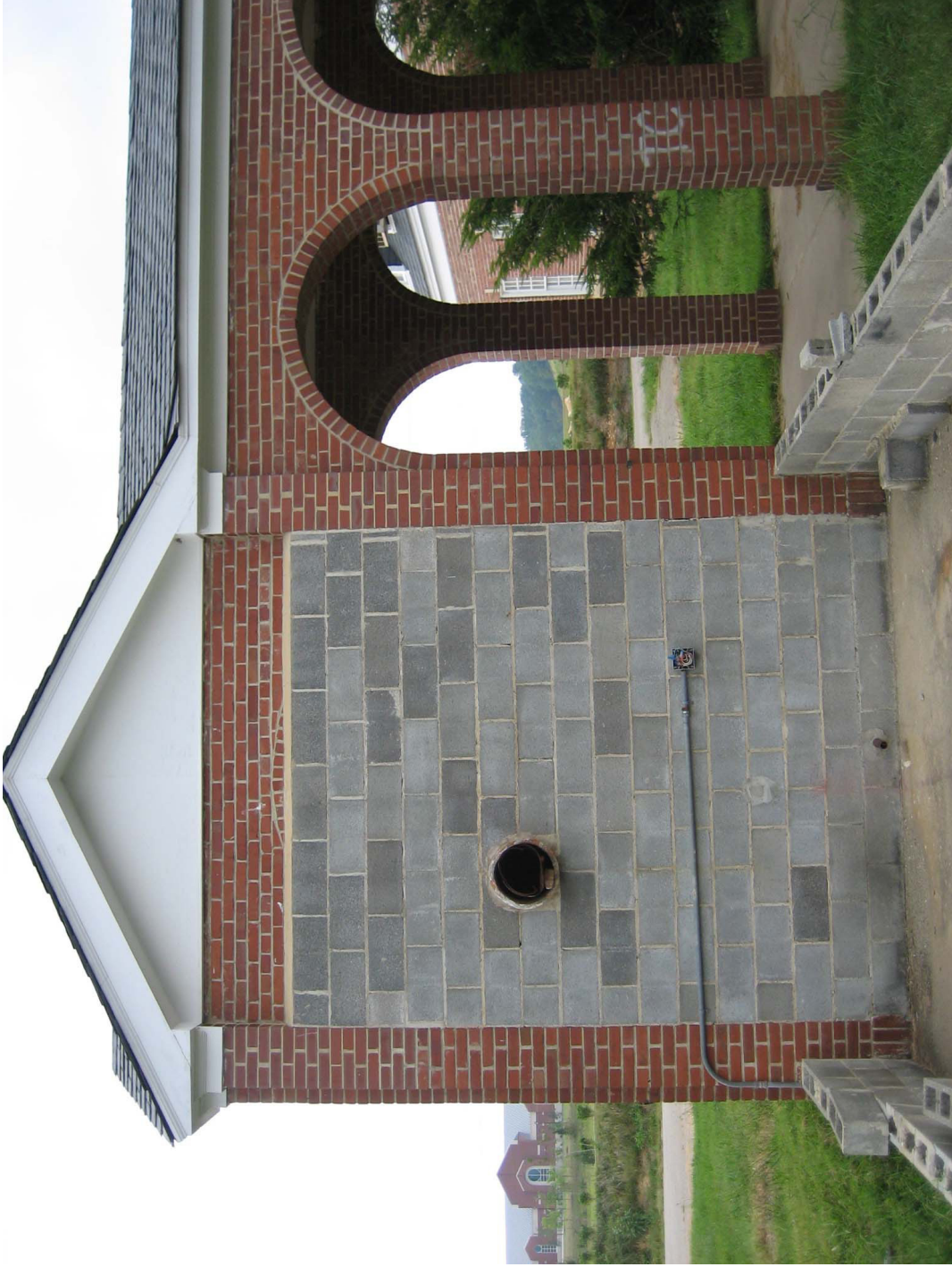
Figure 13: Improvised infill of the open courtyard added in the 1980's when the Workhouse was upgraded to a medium security facility. Photo courtesy of Bruno Grinwis, BBGM architects.
