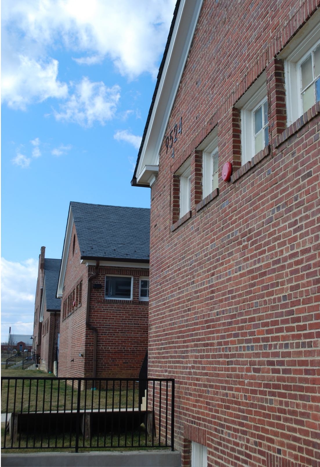
Figure 22: Rear view of prison dormitories renovated into artists studios and classroom space. Photo by author, 2009.
