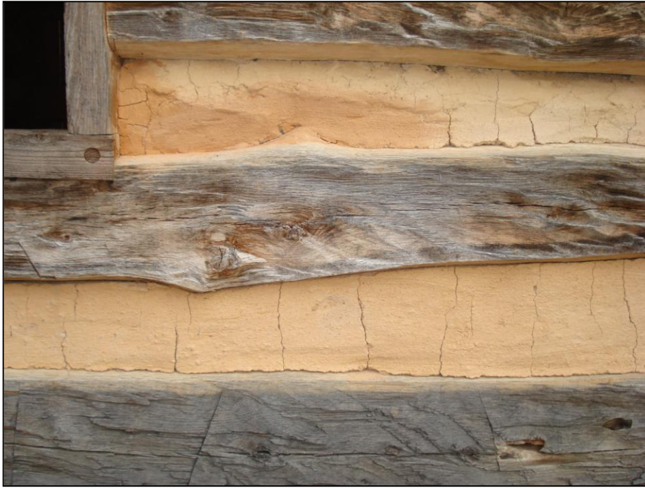
Fig 3.9. Lauren Knight, Detail of Exterior of Log Cabin, Planks and Chinking . 2010. Photograph. Alexandria, Virginia.
