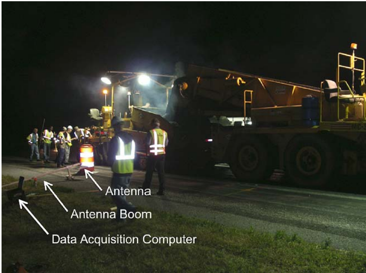
Figure 5.5 – Paving operation and test set up during construction
