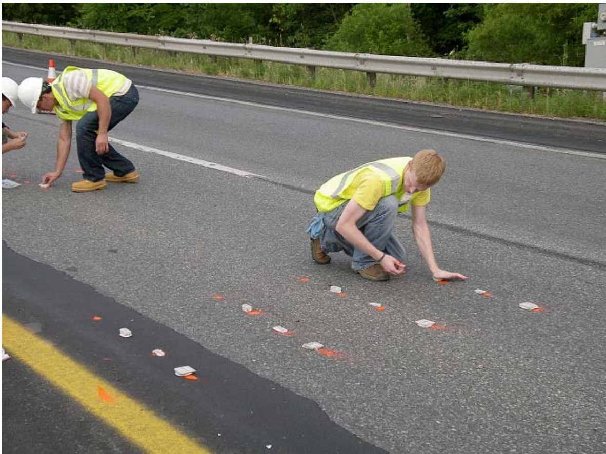
Figure 5.4 – Placement of SAW RFID tags on surface of existing milled pavement
