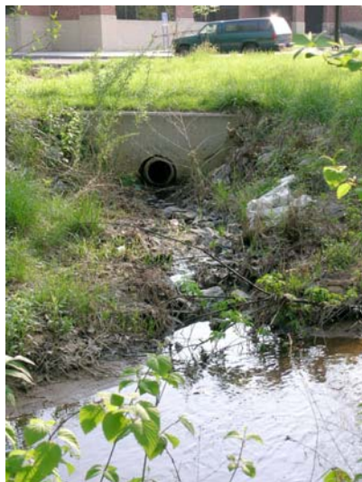
Figure 2.XX Storm water culvert draining the parking lot north of the Agriculture/ Life Sciences Surge Blvd. (Author) Figure 2.XX Looking west across Paint Branch Creek to the point where Campus Creek flows into it. (Author)
