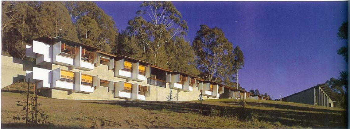
Figure 4.XX East façade with the sleeping quarters in the foreground. (Beck)
