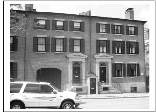
Benefit Street row homes. One of the few examples of row homes in Providence
