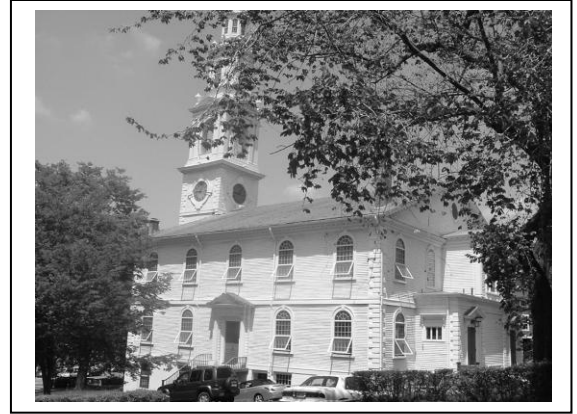
First Baptist Church, at 75 North Main. Side view.
