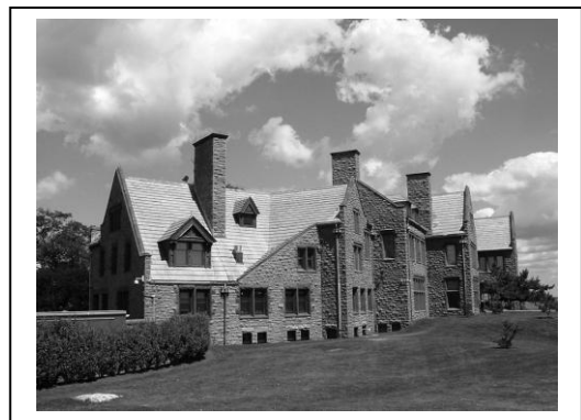
Contemporary Rough Point, viewed from its cliff side.
