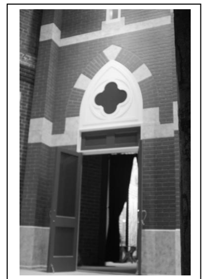
Full-scale exterior of the Church exhibit
