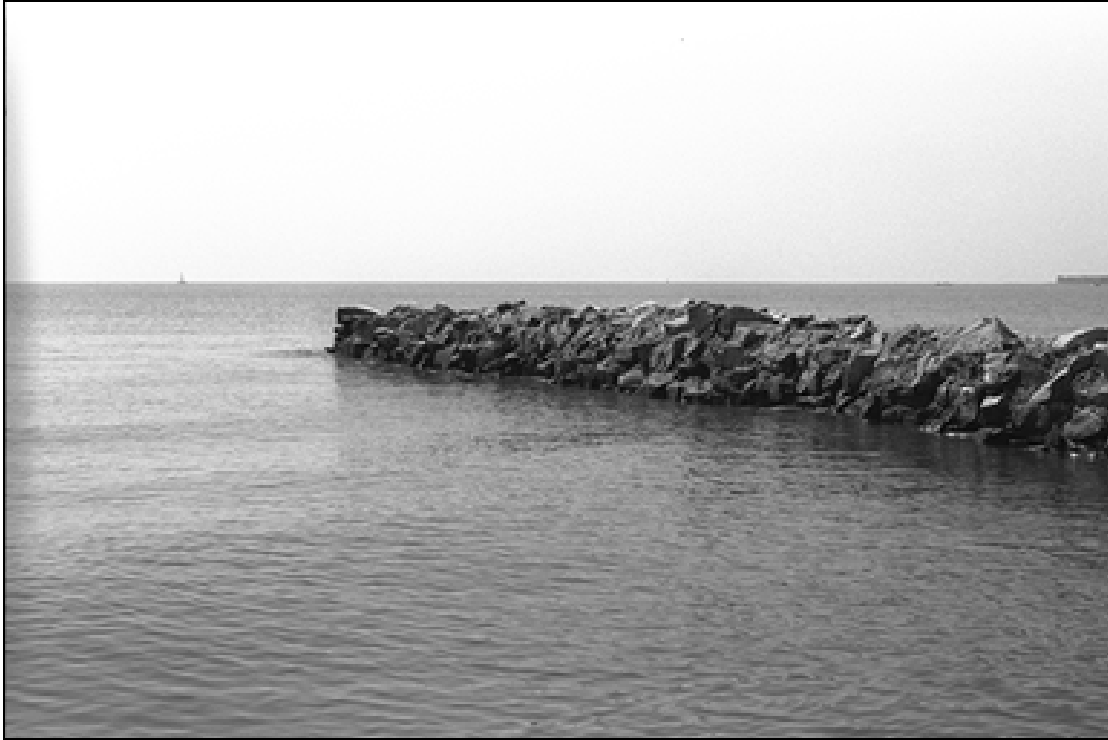
Figure 45: Stone Breakwaters along the Chesapeake.
