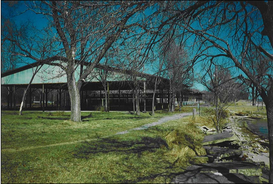
Figure 21: Photo of Remnants of Steel Buildings.
