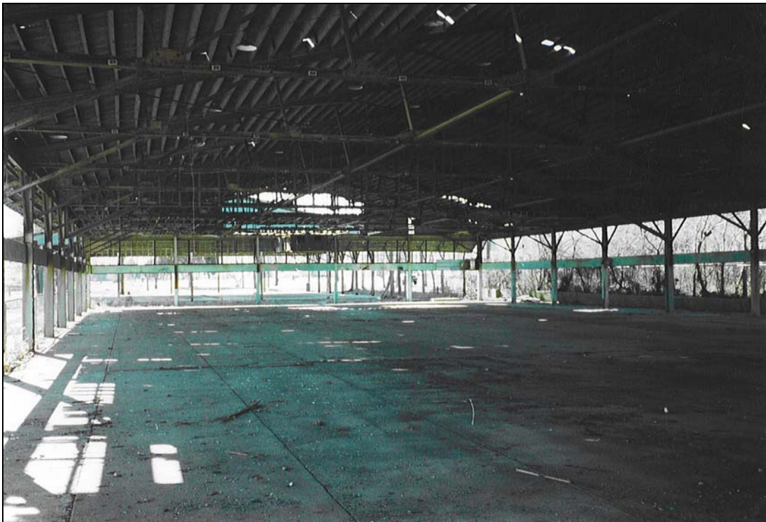
Figure 22: Photo of Inside of Old Steel Buildings.
