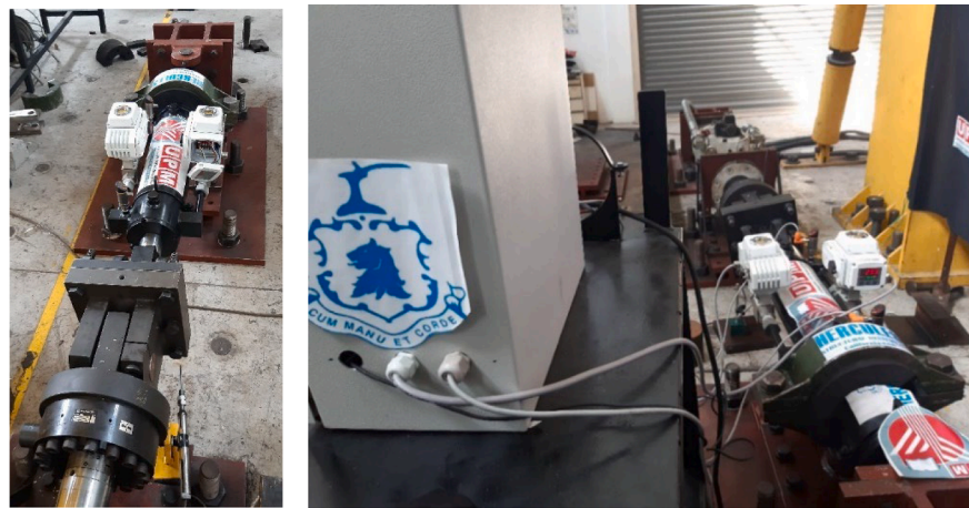
(a) Installed SABFD damper (b) Connection to the PLC controller
