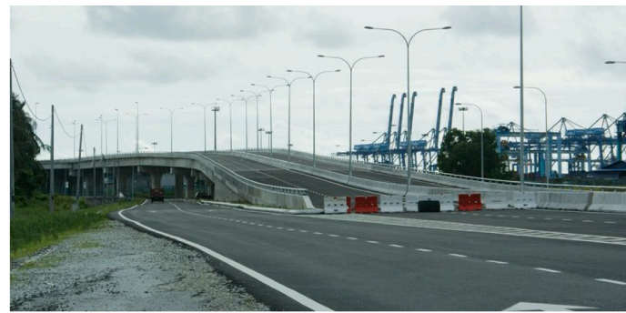
Lebuhraya Pulau Indah bridge in Malaysia
