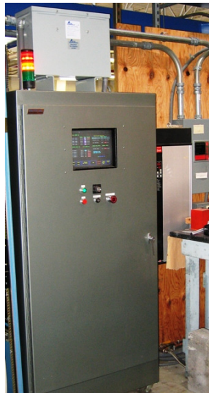
Figure 3.24 The FACTS control system was used mainly to control the temperature and the screw speed of the extruder.
