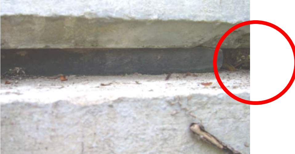
Figure 3.6 - Beginning Stages of Creep
