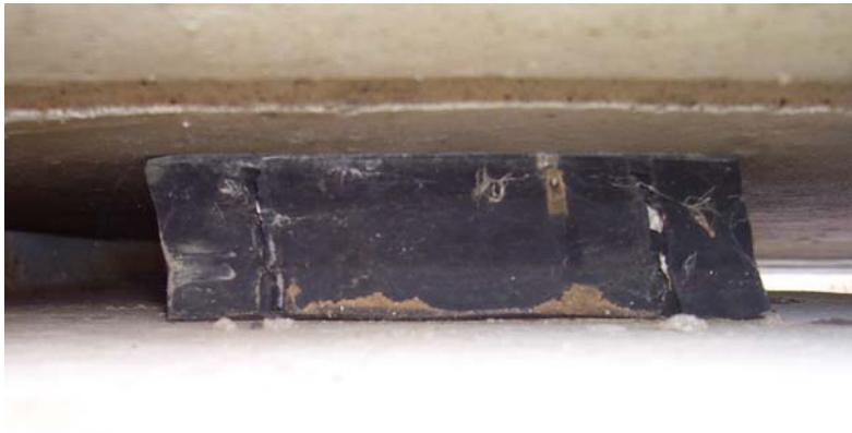
Figure 3.7 - Bulging in a Laminated Bearing
