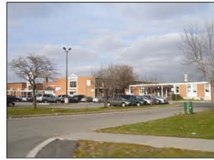
2 - Central Peel Public Secondary School
