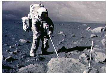
Figure 3-2: Jack Schmitt Using Scoop [29]
