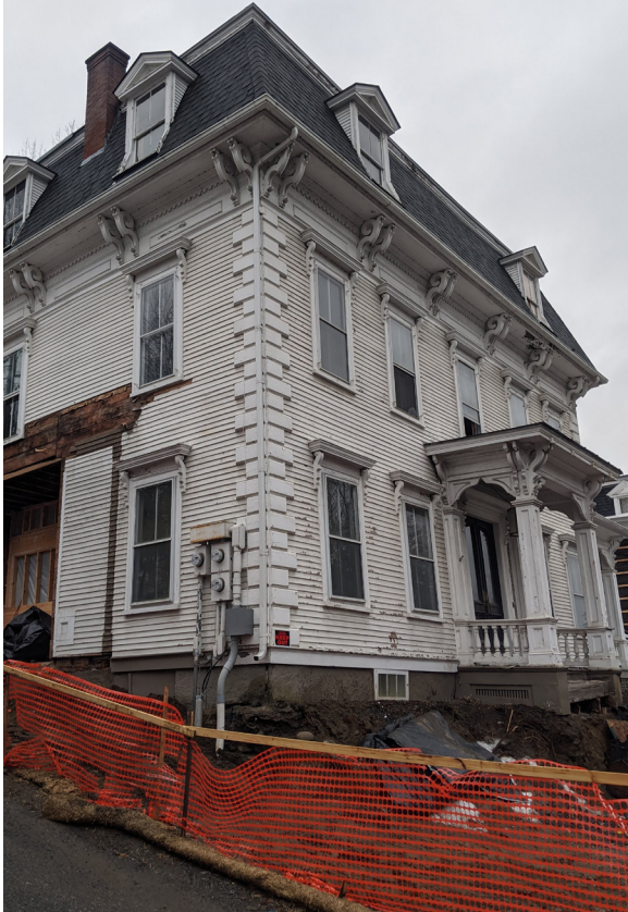
Old home awaiting restoration work in Woodstock, VT
