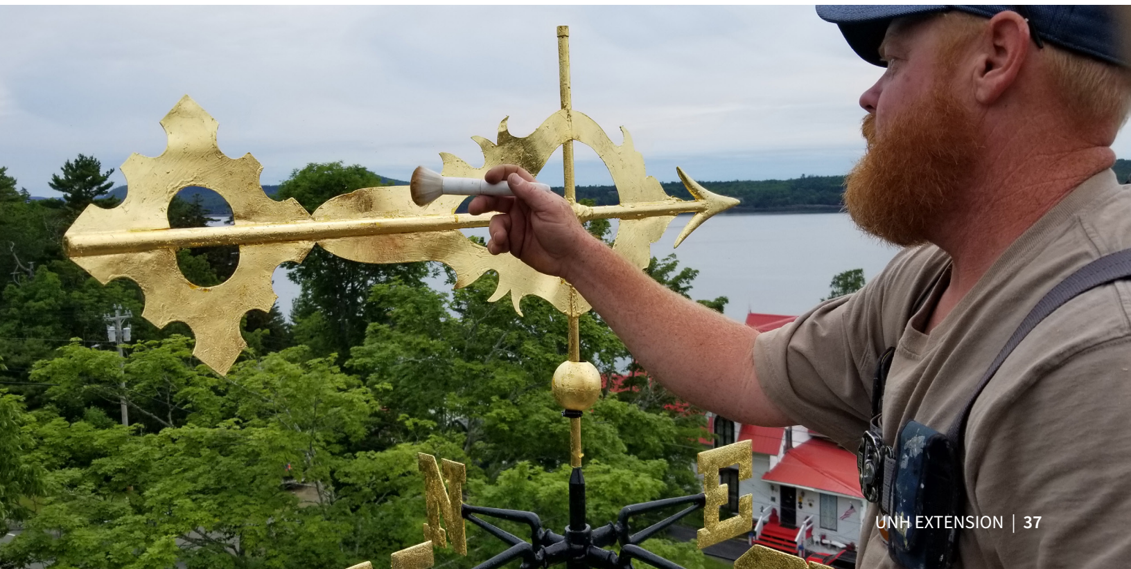
Mid-Maine Restoration finishing the weathervane on the Sewall Memorial Congregational Church, Robbinston, ME. Photo: Maine Preservation.
