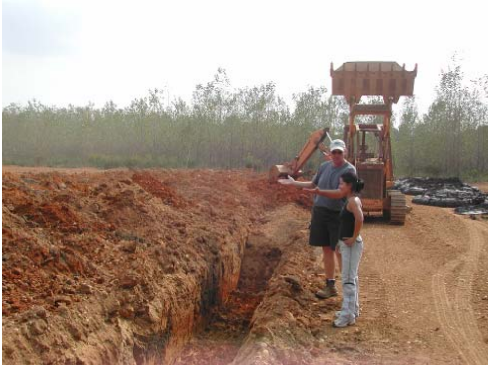
Figure 18. Excavated trench (foreground) in preparation for biosolids (background).
