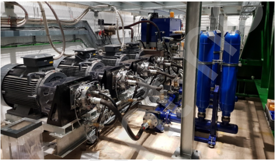
230 231 Figure 4. . FastBlade's Digital Displacement hydraulic pumps.
