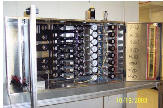
Figure 6. Gas box and its components.
